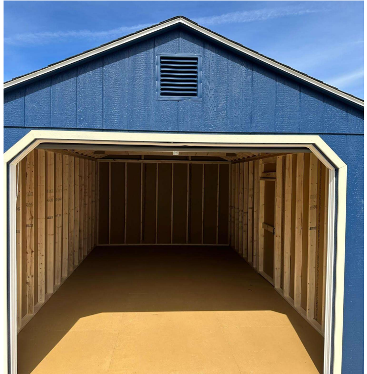
Storage Shed – North Star
