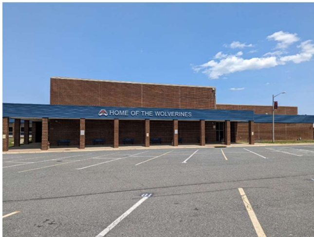
External facade & envelope – North Stafford HS
