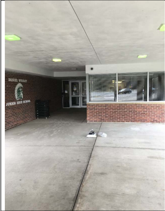
Alternate view outside Subject Building, location for Sample 24026015.
