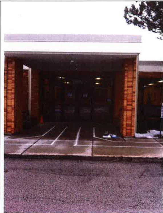
View outside Subject Building, location for Sample 21861789.
