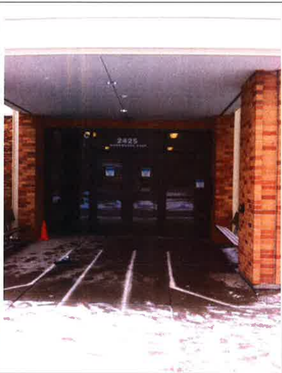
View outside Subject Building, location for Sample 21861841.
