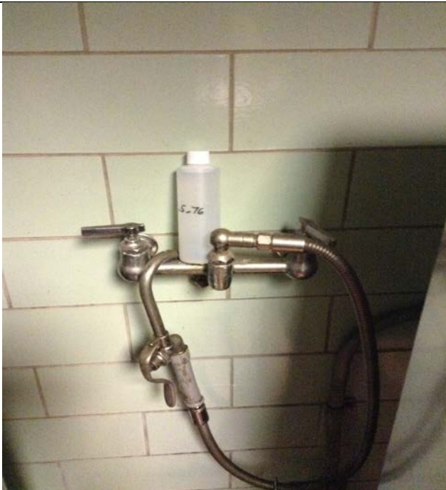
View of Kitchen Spigot Location, Sample #: 448.5-76
