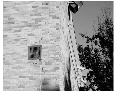
Masonry cracks
