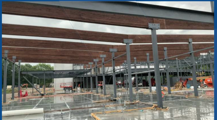
GluLam Beam Install
