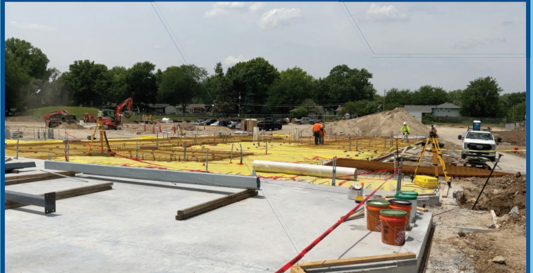
Area B Slab-on-Grade Prep.
