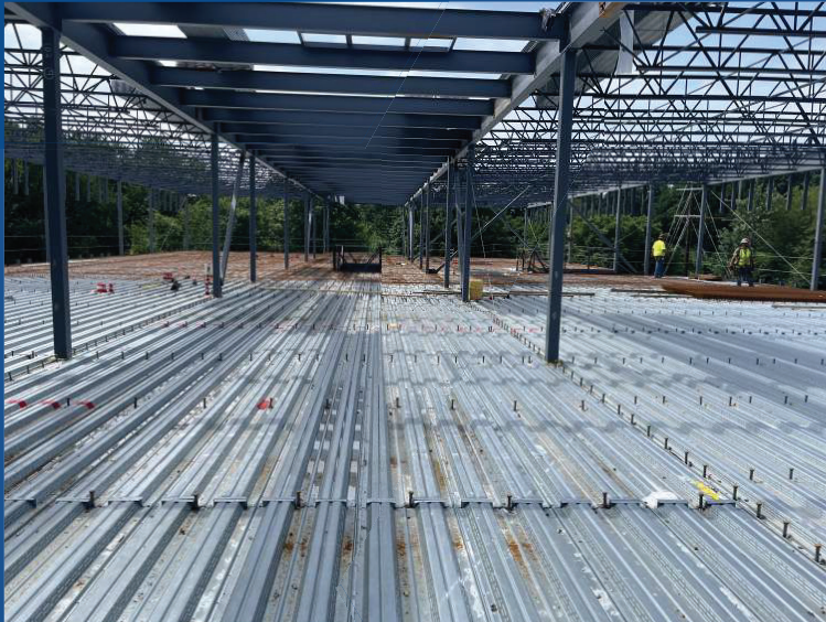
Area D Slab on Deck Preparation
