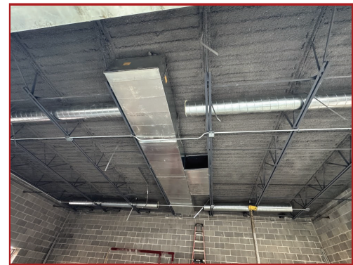
MEP Rough-In at Addition Ceiling
