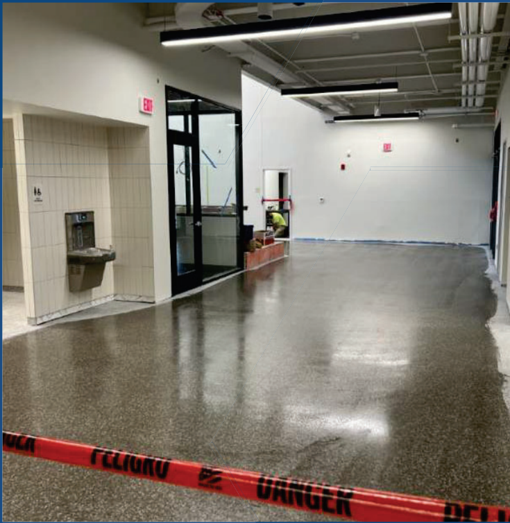
Corridor Concrete Polishing
