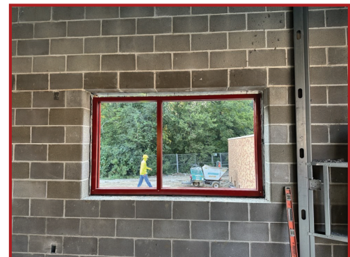
Addition Storefront Window Framing
