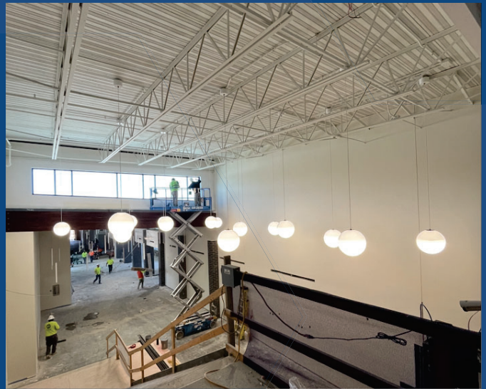
Area C Light Fixture Install
