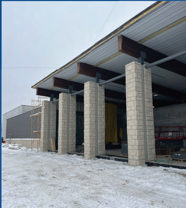
Exterior Masonry & Stone Install
