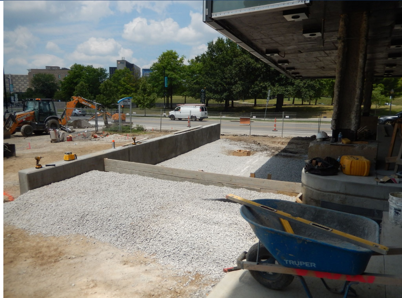
Entry concrete retaining wall
