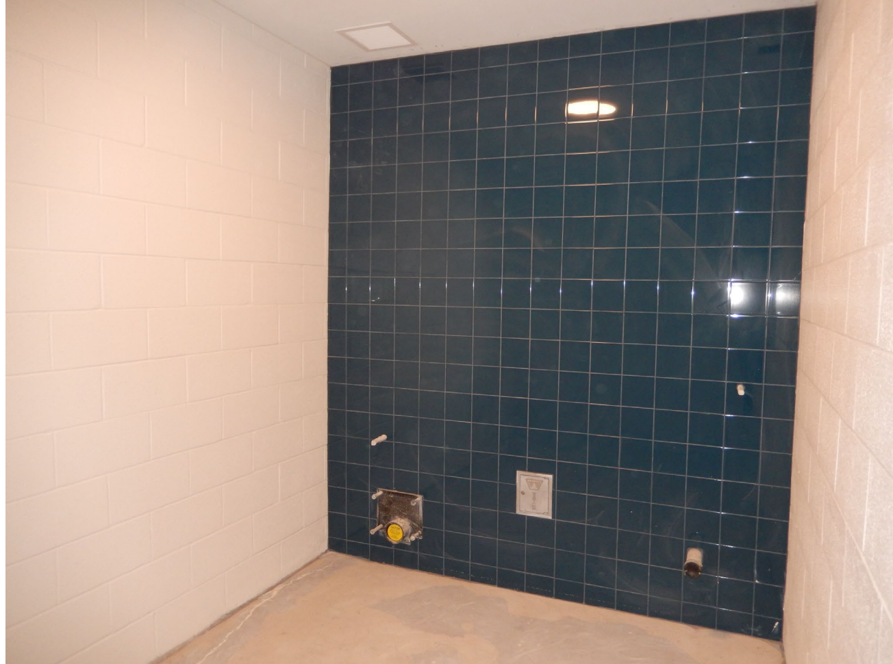
Ceramic tile in Level 3 restroom
