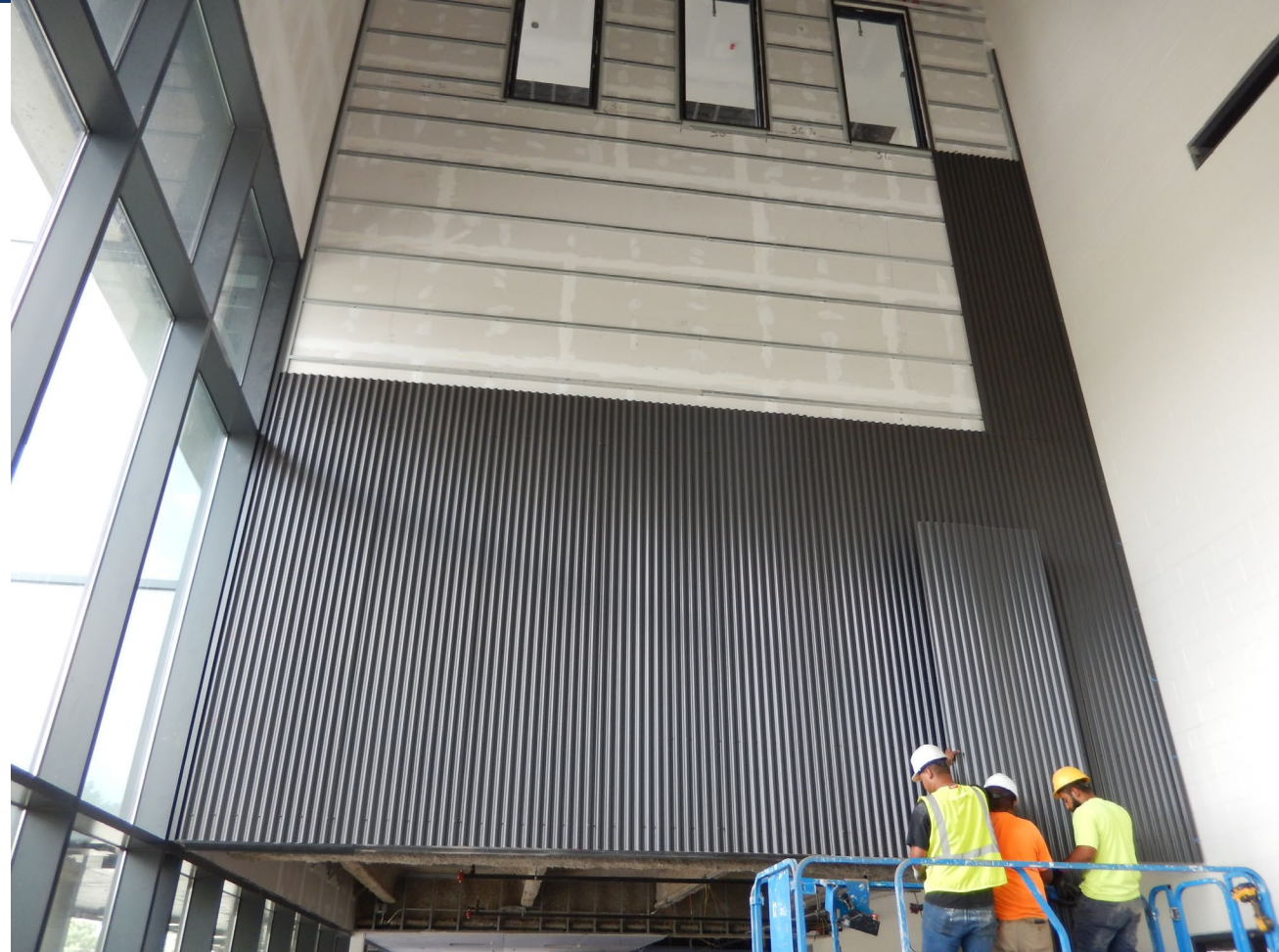
Metal panels at Commons Area
