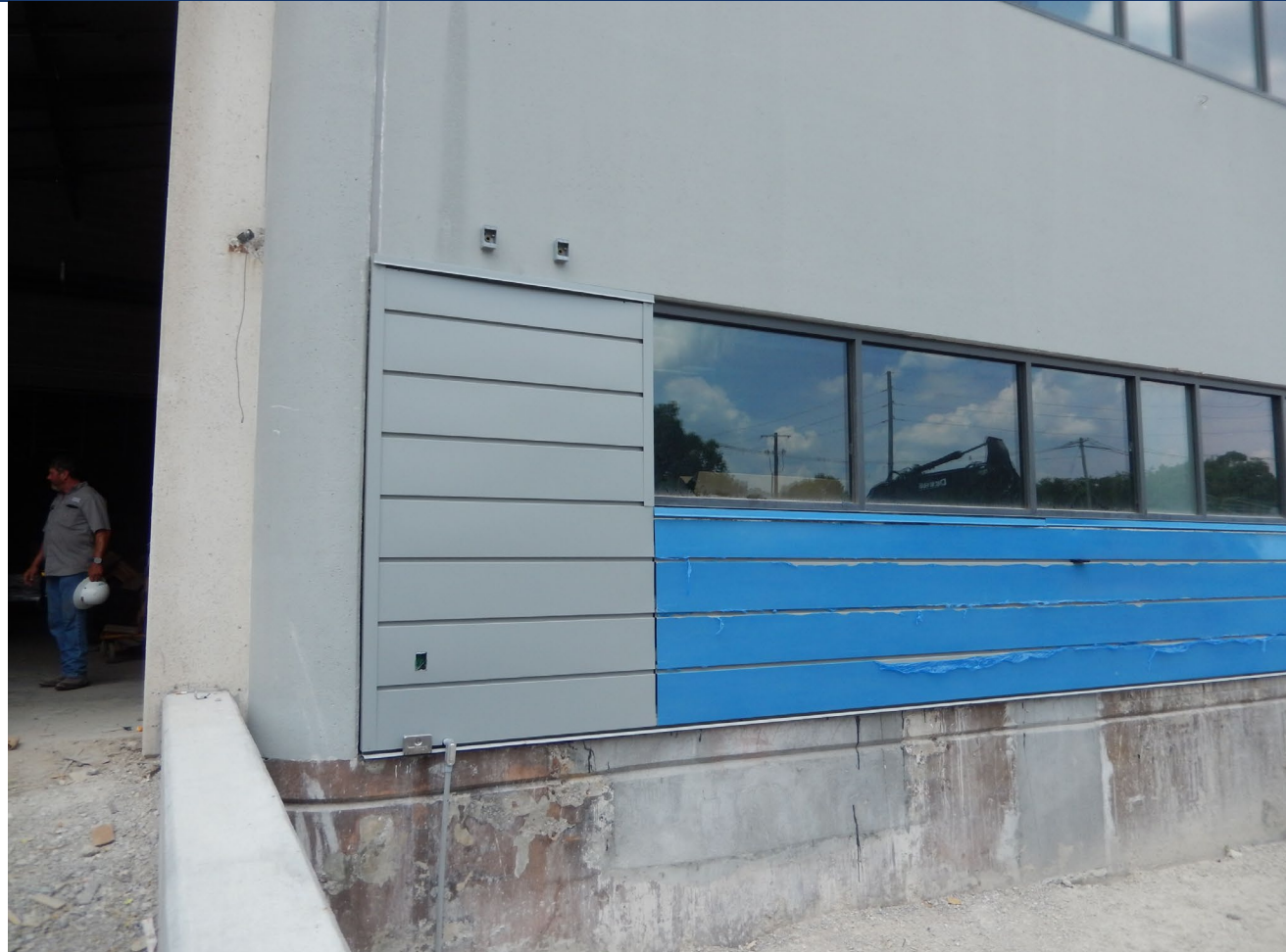
Metal panel at rear of the building
