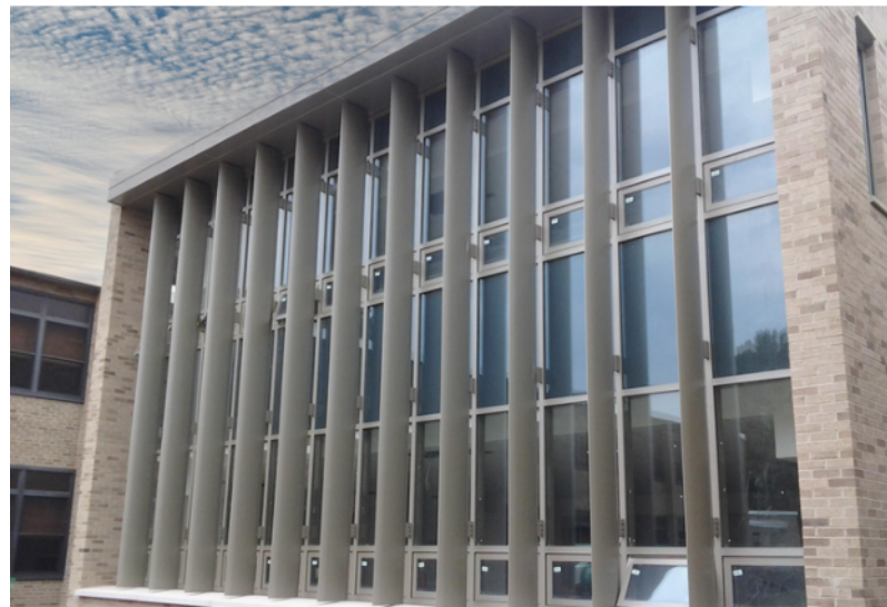
B. VERTICAL BLADES ATTACHED TO MULLION
