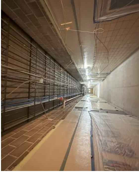
Ridgeview - Hallway Ceiling Demolition
