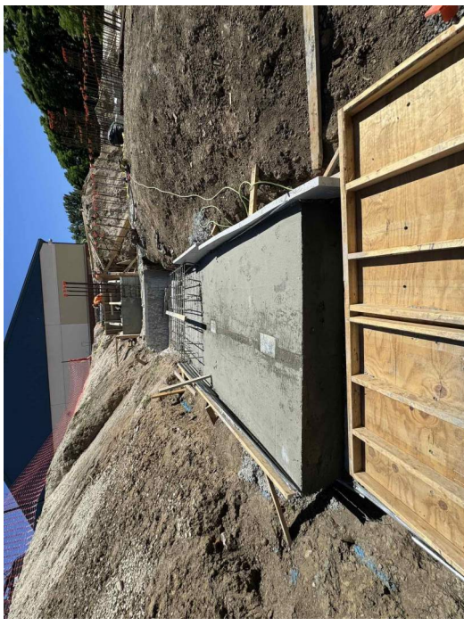
EPiC Elementary - Footings
