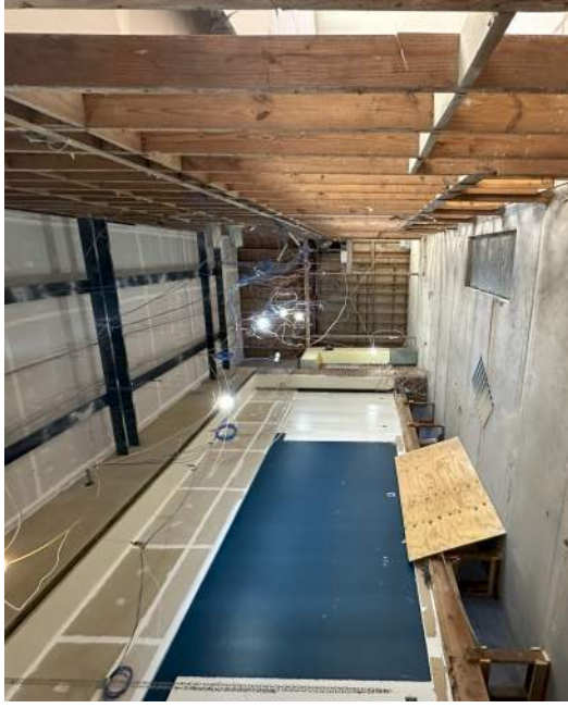
Franklin - Stage Demolition
