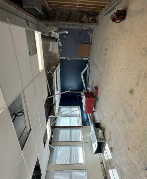
Franklin - Admin Office Demolition
