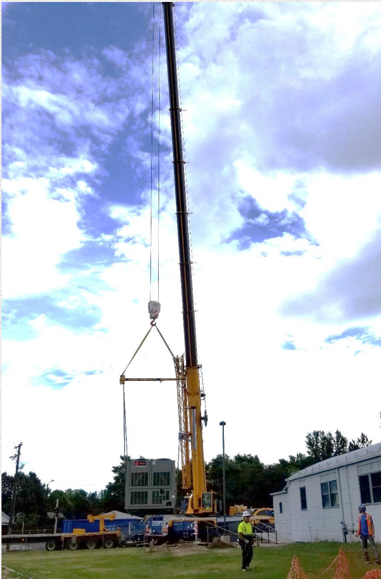
Installation of A/C
