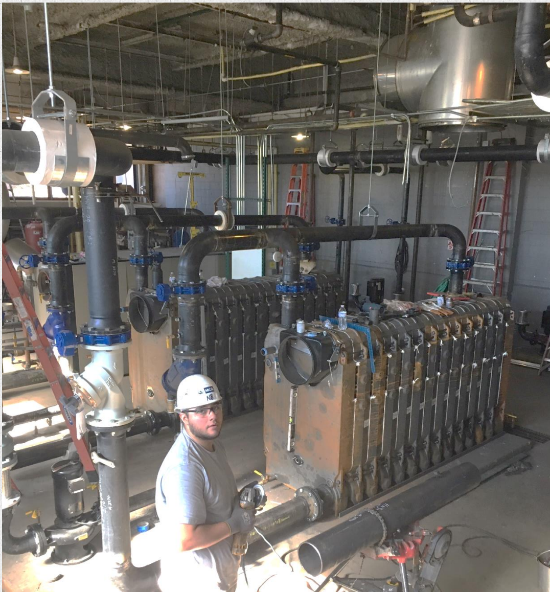
Coronado High School – Boiler Replacement and Upgrades $1,300,000
