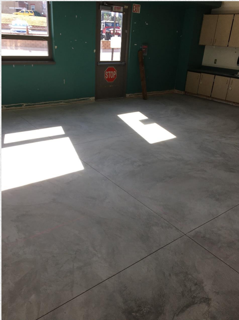
McAuliffe Elementary School – Structural Repairs $150,000
