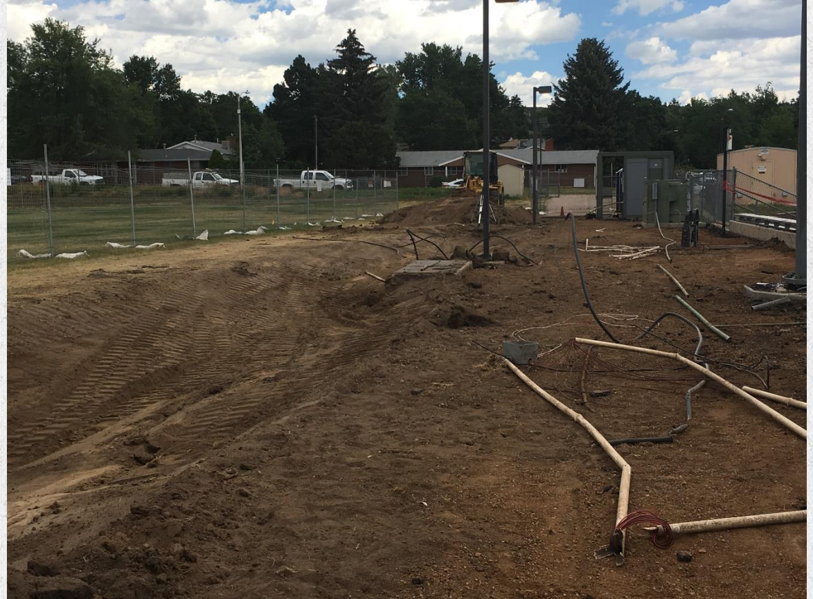
Garry Berry Stadium – Drainage Improvements $175,000
