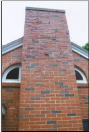
Chimney with significant deterioration, with brick shifting and cracking.
