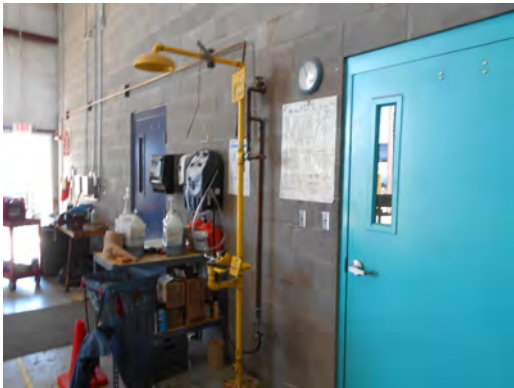
Canutillo_Facilities_Transportation Safety Shower
