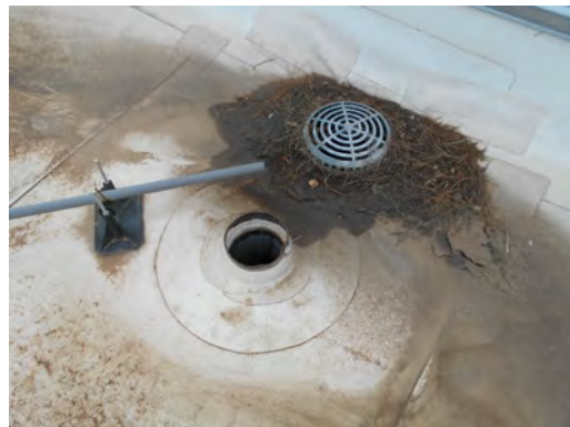
Damian_ES Roof, clean debris and install drain debris covers
