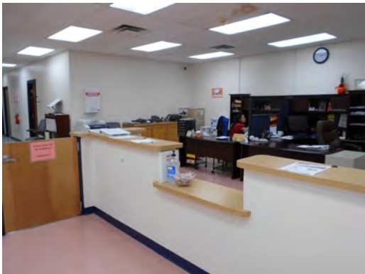
Canutillo_Facilities_Transportation Countertop not ADA compliant
