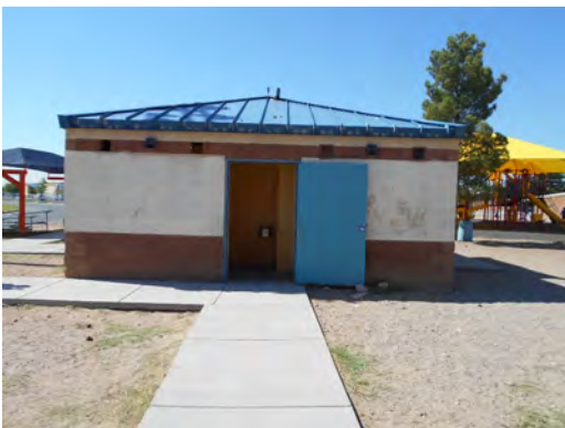
Canutillo ES_Repaint exterior door
