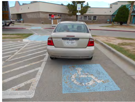
Damian_ES Parking lot deficiency, restripe
