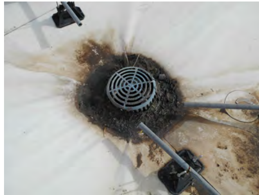
Alderete_MS Main Building, clean and clear debris from roof
