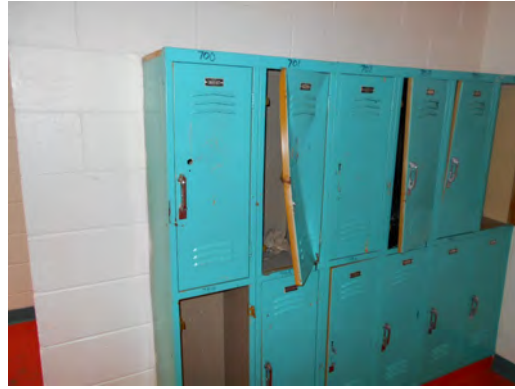
Alderete_MS Main building, replace old damaged locker system
