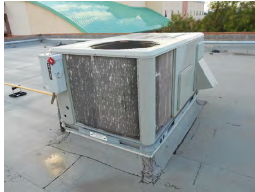
Alderete_MS Main building, replace old RTU's
