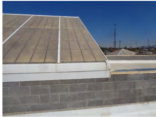
Canutillo ES_Seal CMU wall and recaulk parapet wall joints
