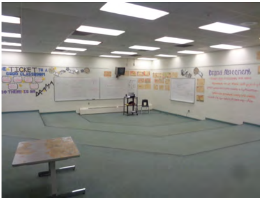
Alderete_MS Main building, replace old worn carpet
