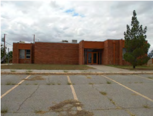
Canutillo_MS Former Admin Bld B, abandoned
