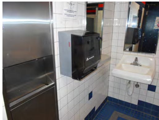
Canutillo_MS Replace paper towels with hand dryers
