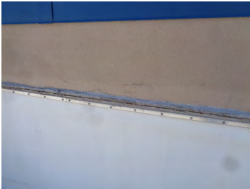
Davenport_ES Parapet wall seal and caulk joints
