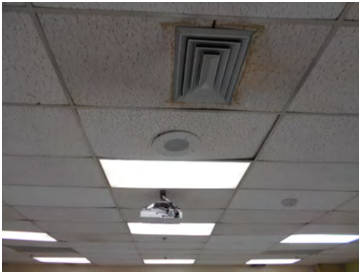
Canutilo_MS Replace old ductwork and registers
