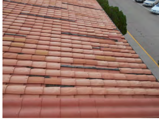
Lone_Star_Buildings Unused Bld, roof
