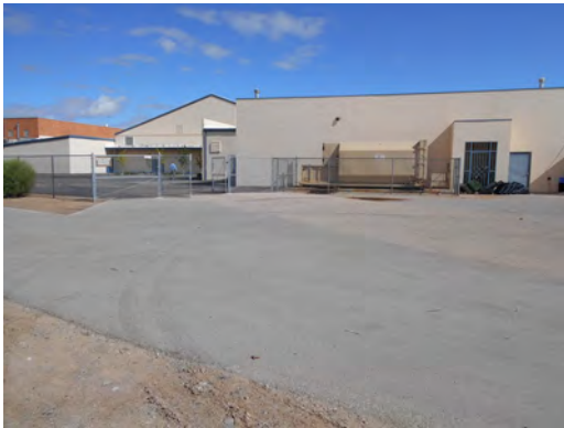
Canutillo_MS Parking Lots, repave and restripe
