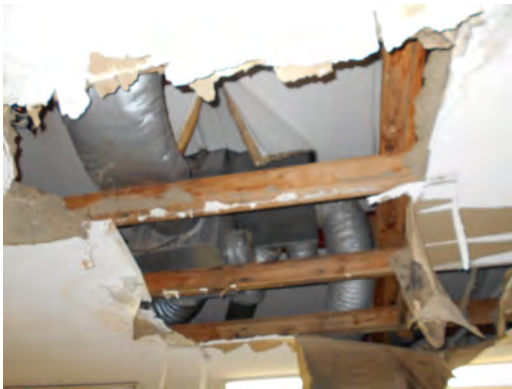
Canutilo_MS Warehouse interior ceiling
