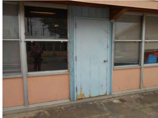
Lone_Star_Buildings Main Bld exterior doors
