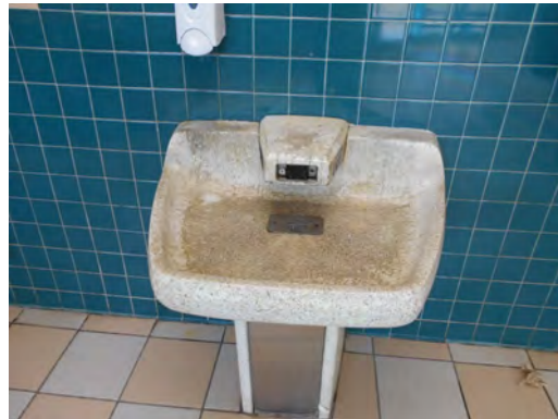
Damian_ES Replace non working restroom lavatory
