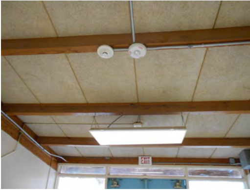
Lone_Star_Buildings Main Bld, Tectum deck
