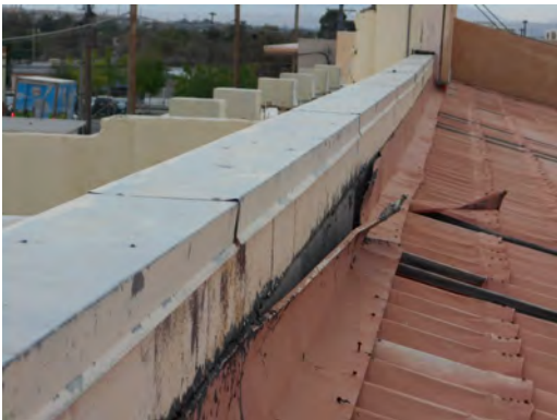
Lone_Star_Buildings Unused bld, roof
