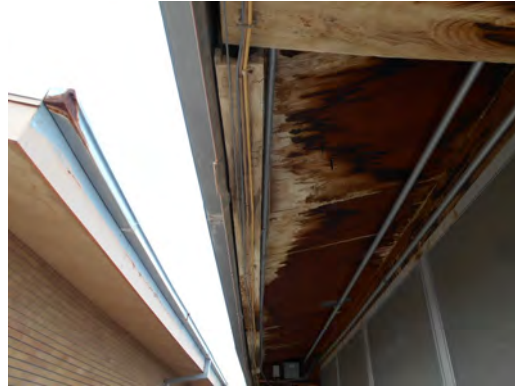
Lone_Star_Buildings Main Building soffit
