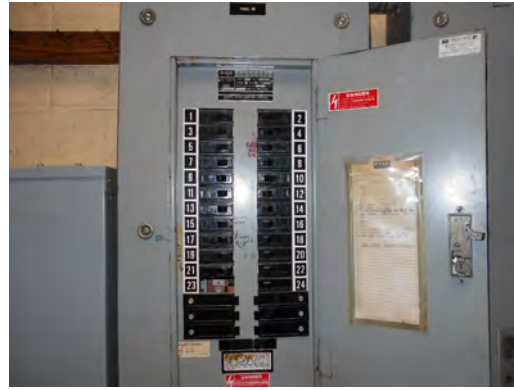
Alderete_MS Main building, replace all old Federal Pacific electrical panels
