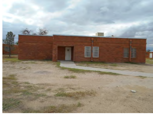
Canutillo_MS Former Admin Bld A, abandoned
