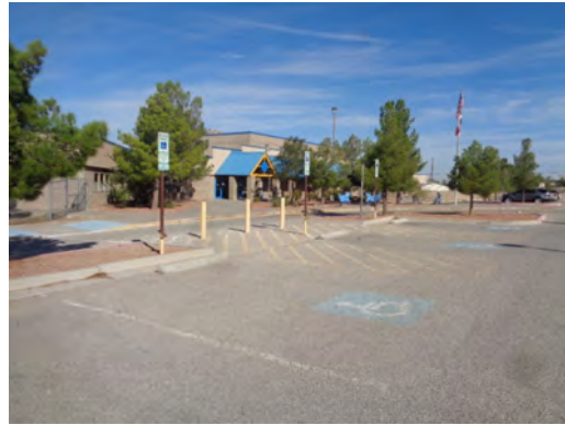
Davenport_ES Parking lot repairs and restripe
