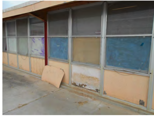
Lone_Star_Buildings Main bld, exterior window/wall system
