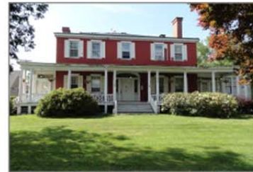
Existing Historic House to be restored
