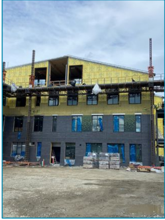
Brick veneer and window installation
