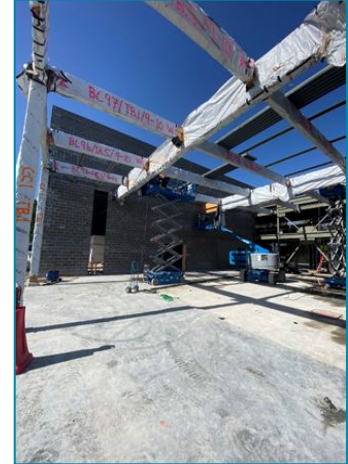
Mass timber beam installation in Creative Arts Studio
