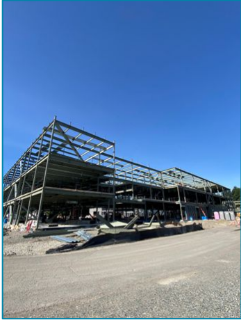
Structural steel erected and concrete slabs poured
