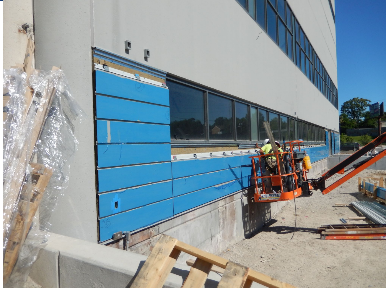
Metal panel at rear of the building
