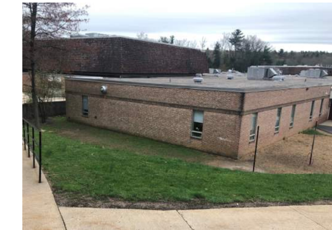
Low area of proposed playground at northeast of building
