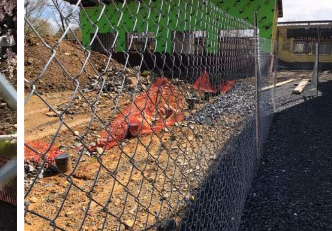
Piping in proximity of proposed mound
