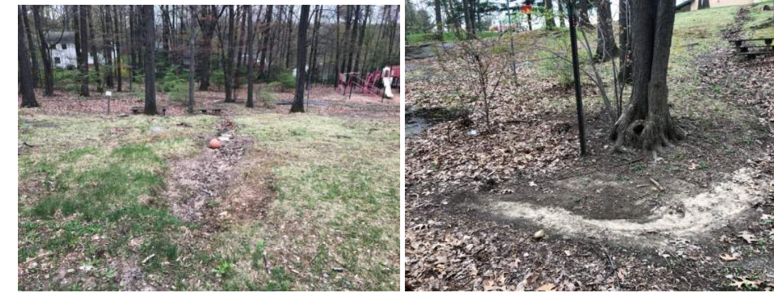
Signs of erosion on hillside
