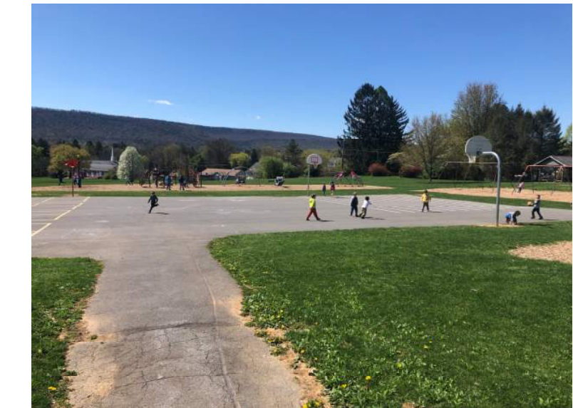
Main asphalt area of existing playground and location of proposed mounded areas
