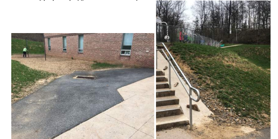
Existing storm grate at NW of bldg.
