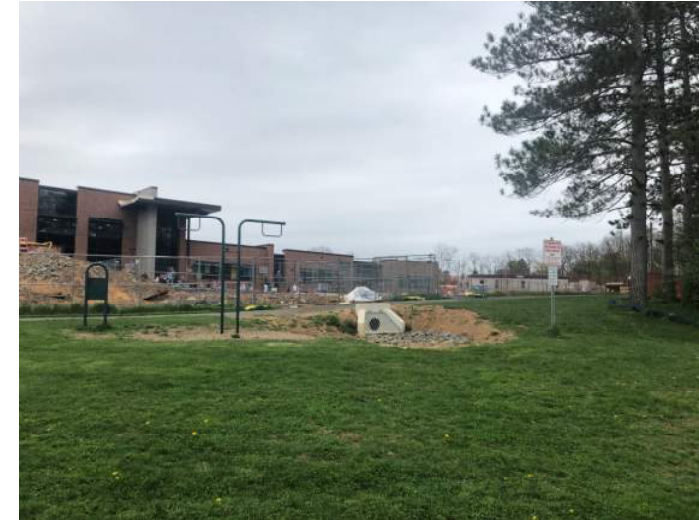
South headwall outflow (note this is within footprint of proposed walkway but beyond existing wooded area)
