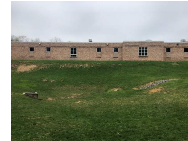
View of basin on the east side of building, facing west
