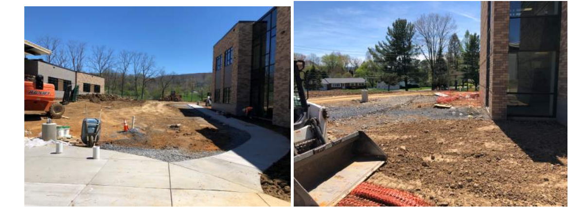
Core area facing east.
