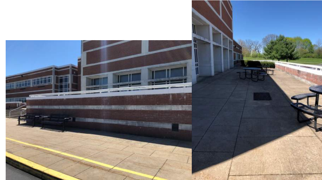
Retaining/half wall of concrete platform area
