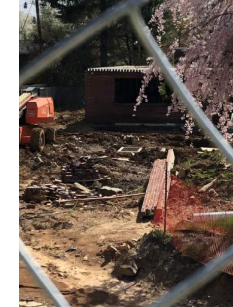
Storm Grate in proximity of proposed mound
