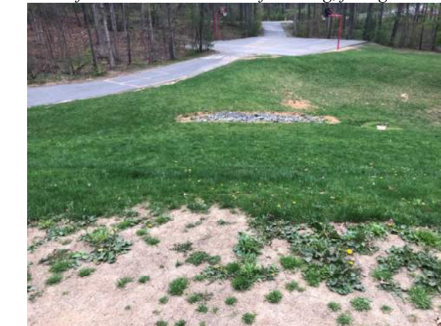
View of basin and wooded area on east side of the building, facing west
