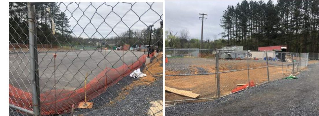
Asphalt play area from bldg. facing southeast
