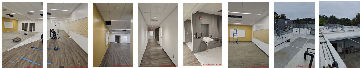
Left to right: various rooms and areas of finish work, from classrooms, restrooms, hallways, to roof with HVAC units in place.
