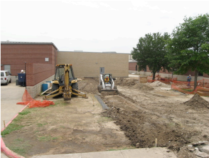
View of sidewalk layout and prep work.
