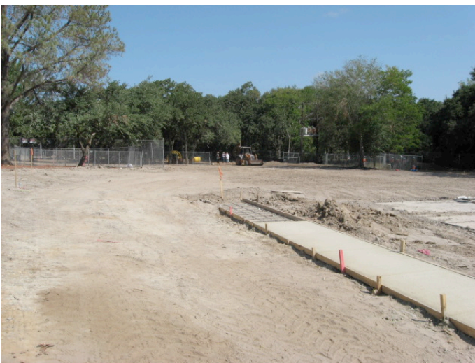
View across the site looking north.
