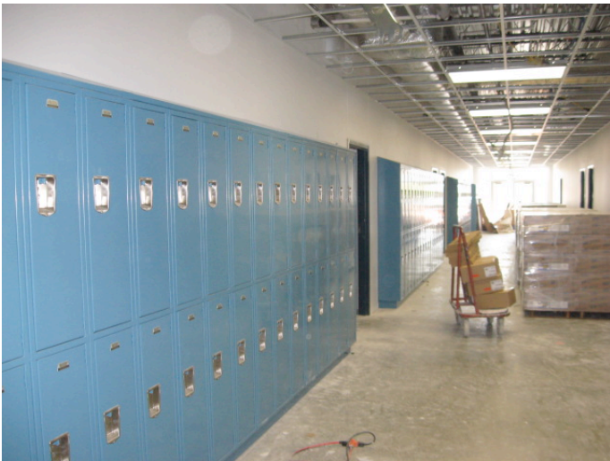
These are the new lockers installed in corridors.
