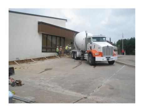
This is the new concrete ADA compliant ramp being installed to the front entry area.
