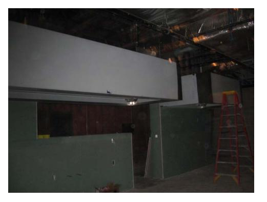
This is a shot of the two massive stainless steel exhaust hoods in the kitchen that were installed this week.
