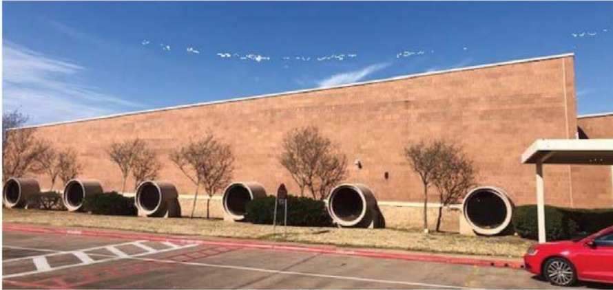
EXISTING EXTERIOR FACADE AT SOUTHWOOD VALLEY ES
