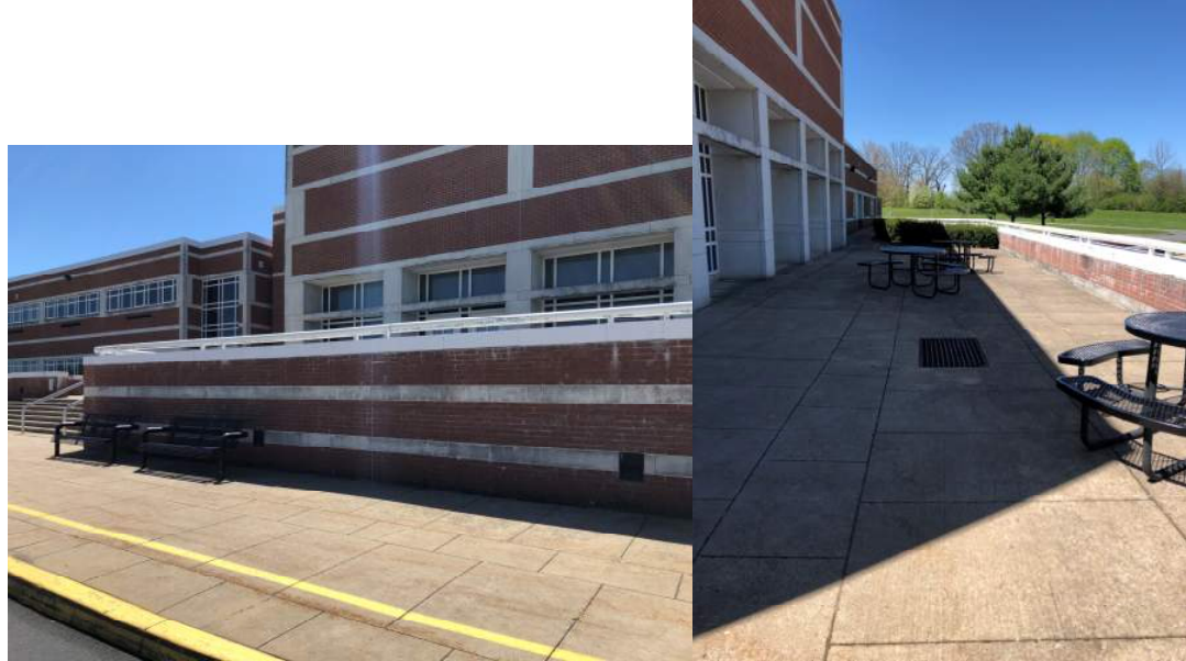
Retaining/half wall of concrete platform area
