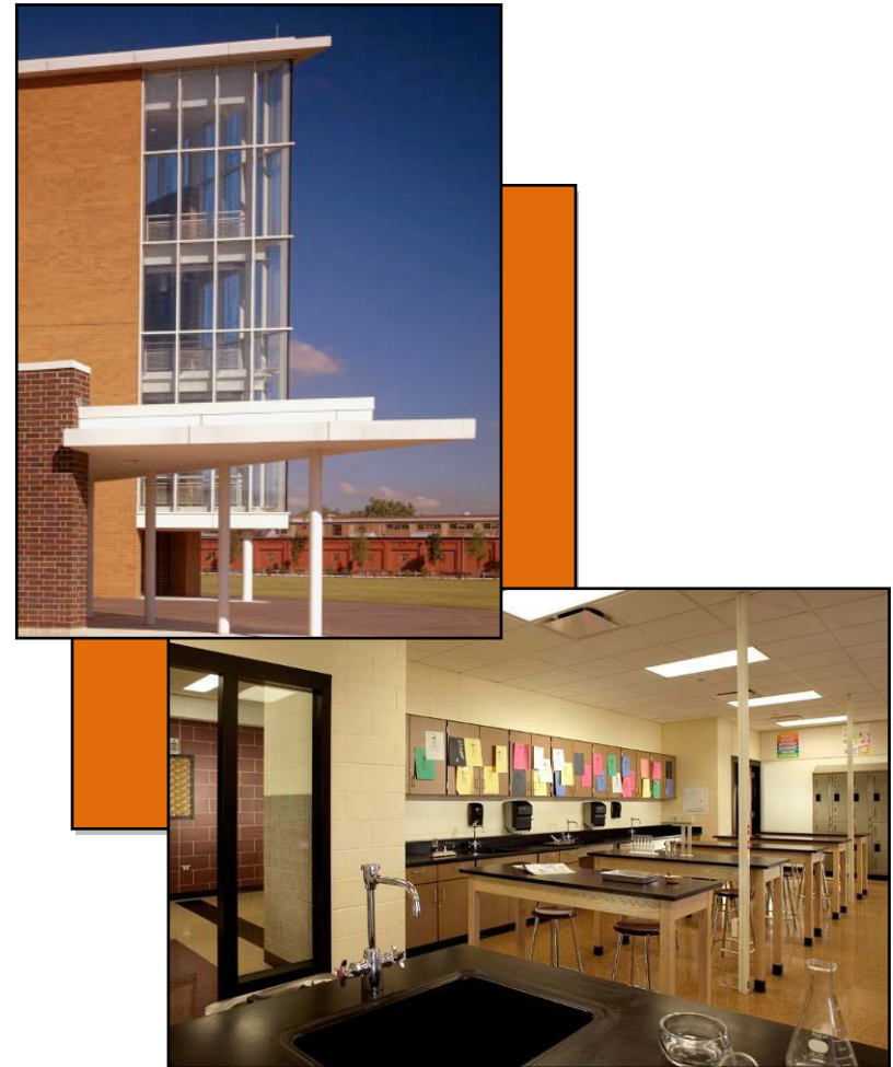
Unity Junior High School, Cicero, IL FGM Architects
