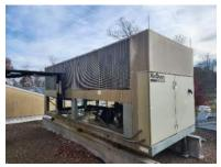
• A McQuay split system chiller is utilized to develop chilled water for cooling. This chiller is original and utilizes R-22 refrigerant. Three of the four compressors are original and have lasted beyond their normal expected lifecycle. R-22 refrigerant has been phased out of production in 2020 due to its ozone
