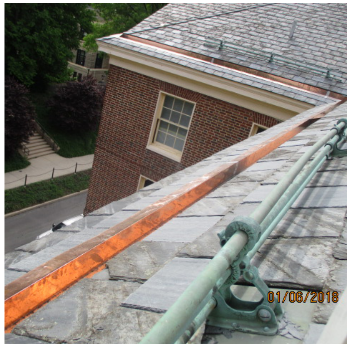
New Copper Gutter Replacement at Hamilton Hall
