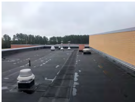
EPDM Roof Membrane
