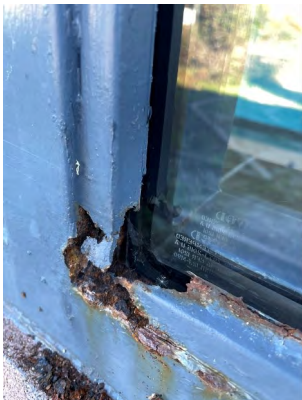
Window Frames in failure
