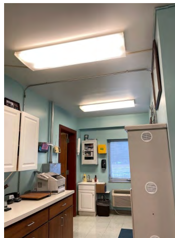
Administration size and outdated finishes
