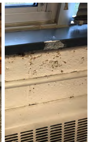
Water Infiltration
