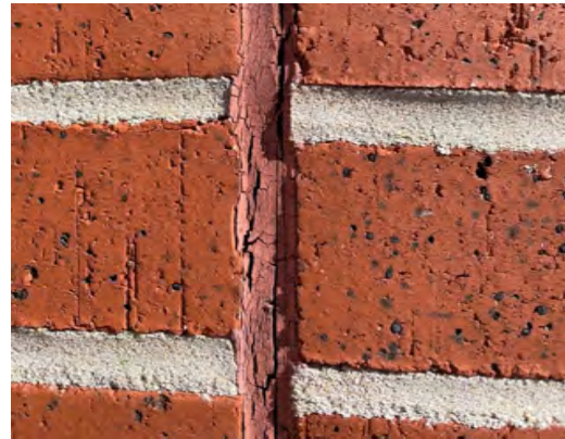
Joint Repairs at Gymnasium
