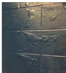
Water Infiltration
