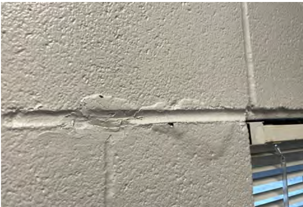
Paint Spalling
