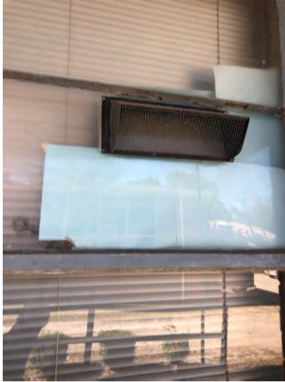
Vent through window
