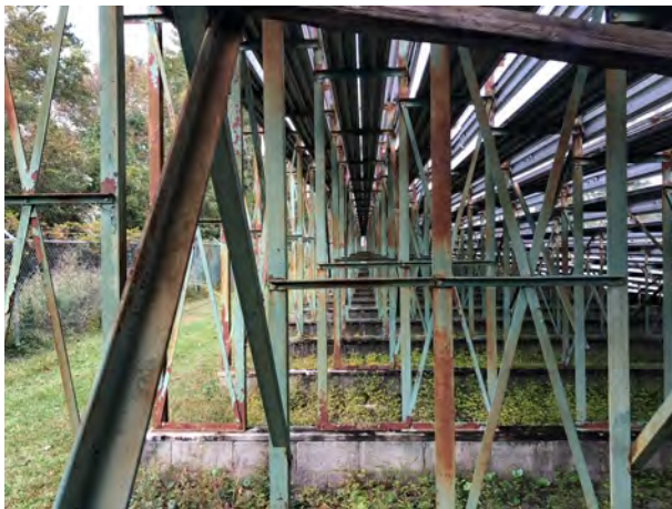
Stadium Structure - paint
