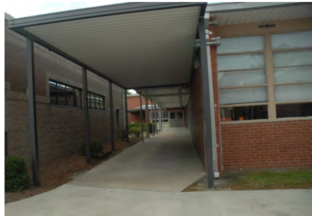
Canopy to older section
