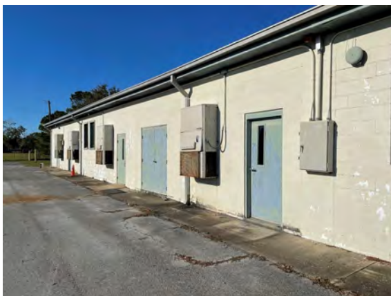
Storage Building at north parking lot
