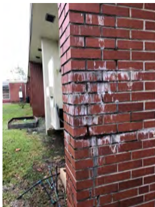
Efflorescence
