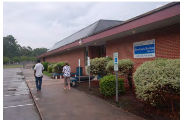
Northwest Entry near Gymnasium
