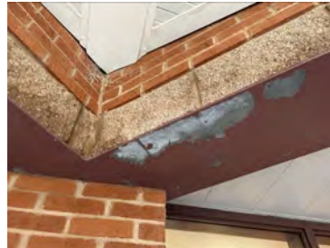
Paint Failure
