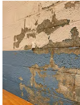
Water Infiltration
