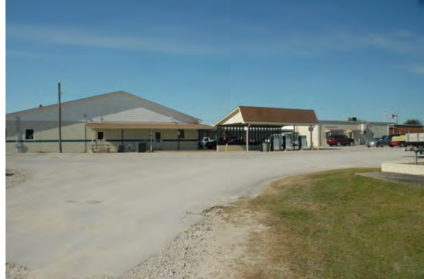
Maintenance / Gas Pumps
