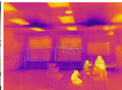
Thermograph with good seals
