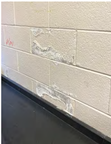
Spalling Paint
