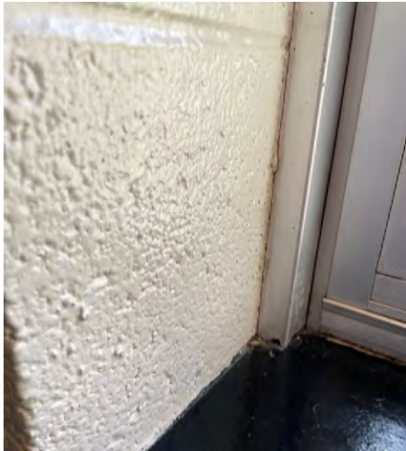
Cinder Block walls
