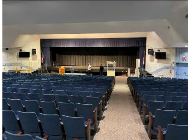
Auditorium in good overall condition
