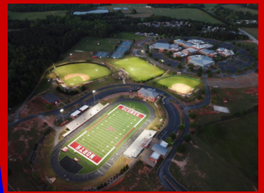
Artificial turf, track, and lighting at Oconee County High School and North Oconee High School
