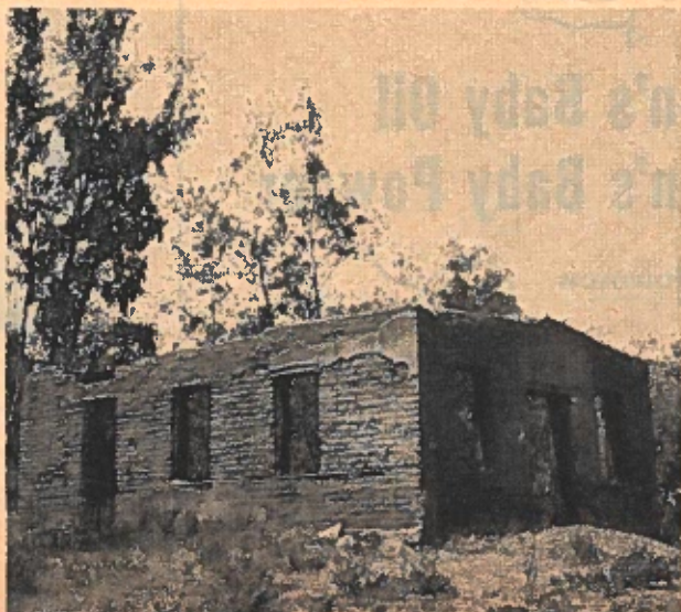
BY 1943 ROOF WAS GONE, ABOVE WALLS BEGAN TO CRUMBLE
