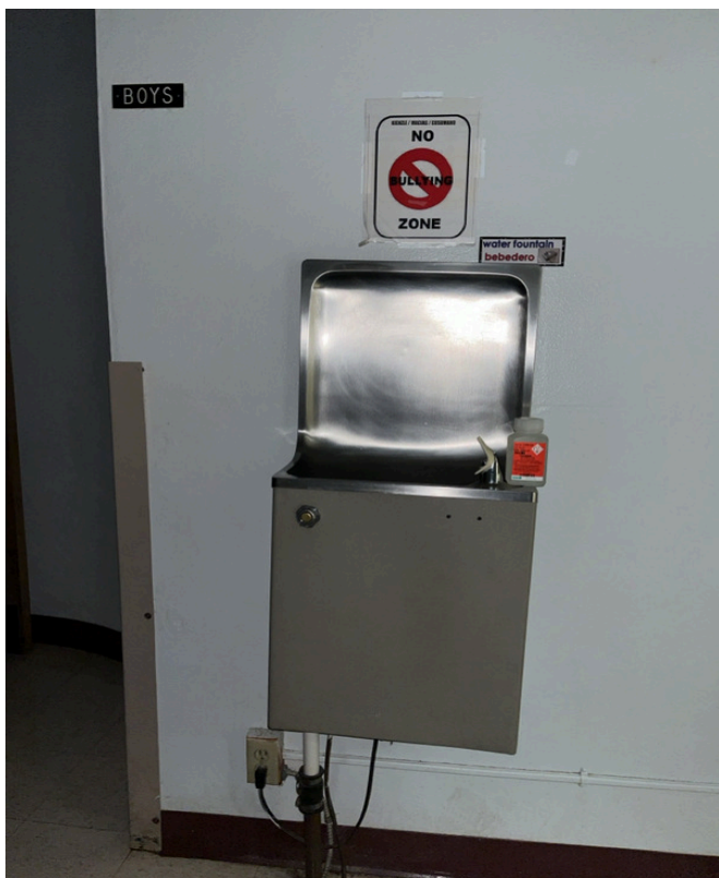
4/9/2024 - 2601-46 - Norclay Building - Outside Men's Restroom
