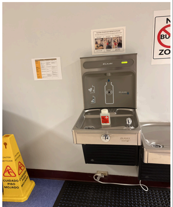
4/9/2024 - 2601-47 - Norclay Building - Outside NC-838-Left
