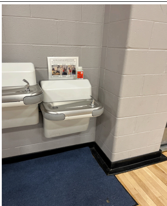
4/9/2024 - 2601-57 - Norclay Building - Gym - Right
