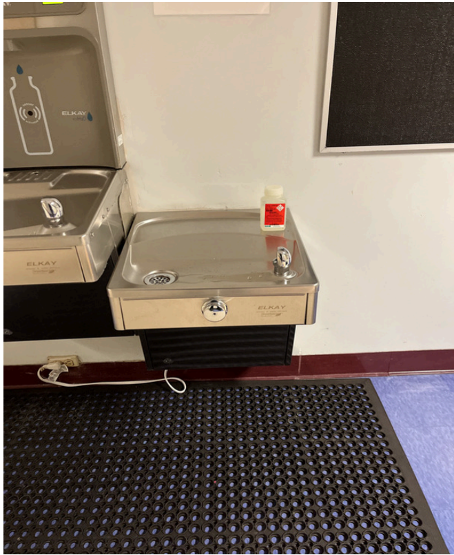
4/9/2024 - 2601-48 - Norclay Building - Outside NC-838-Right
