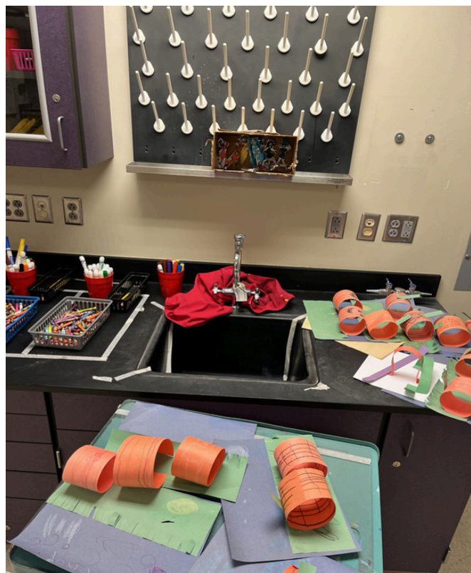
4/9/2024 - 2601-10 - Norclay Building - Room 813 - Northeast - Out of Order
