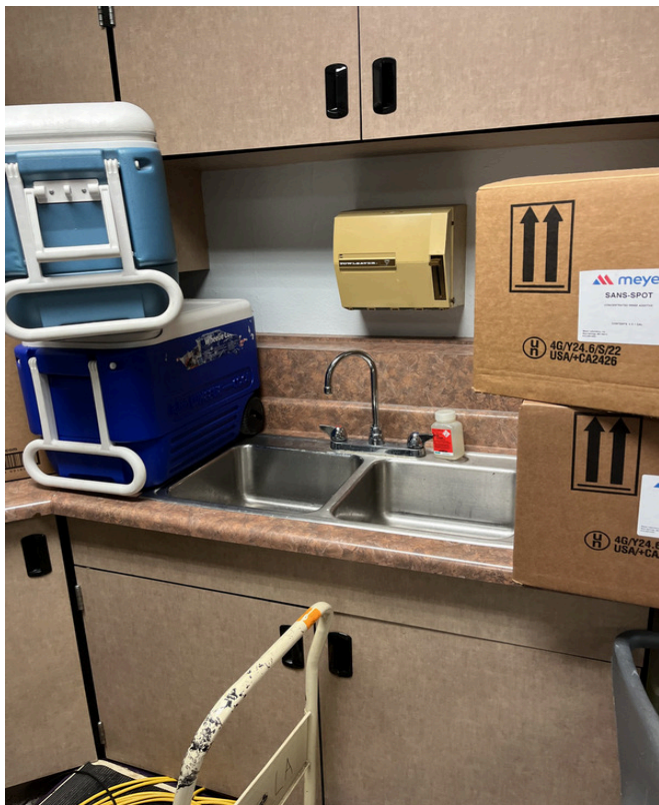
4/9/2024 - 2601-42 - Norclay Building - Room 828 - North Wall Left Sink
