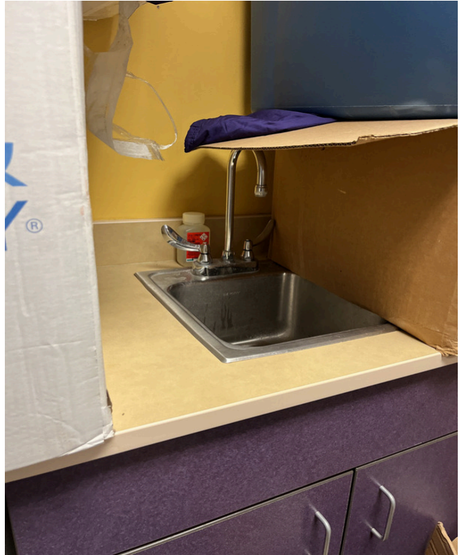
4/9/2024 - 2601-53 - Norclay Building - Room 804
