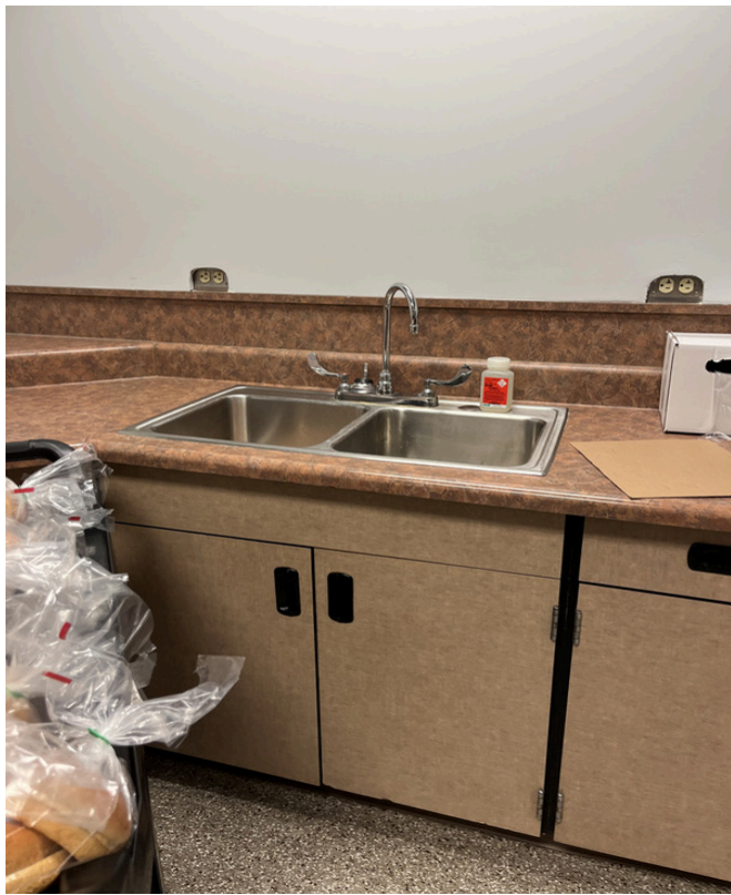
4/9/2024 - 2601-40 - Norclay Building - Room 828 - North Sink
