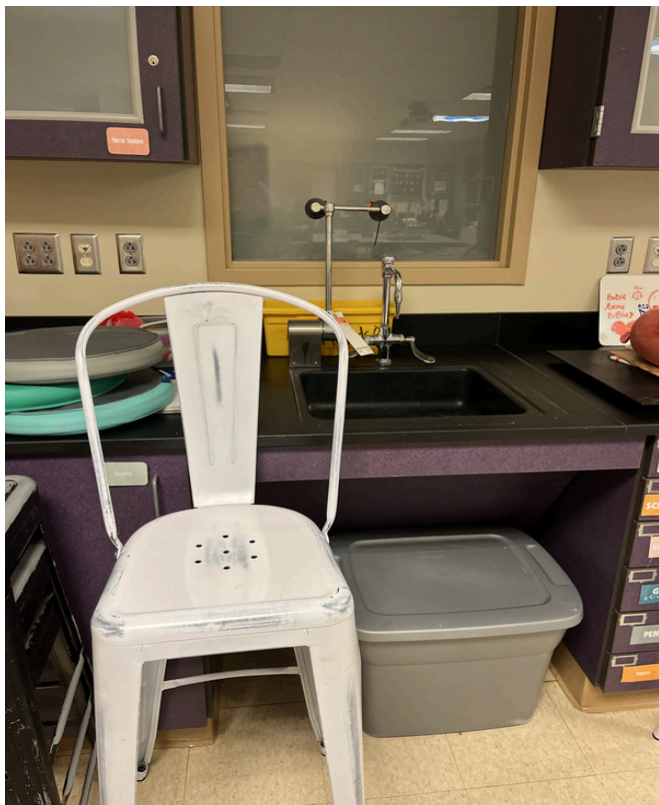
4/9/2024 - 2601-2 - Norclay Building - Room 815 Northwest-Out of Order
