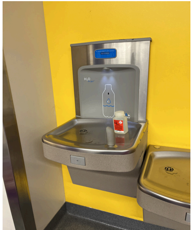
4/9/2024 - 2601-51 - Norclay Building - Wrestling Room - Left
