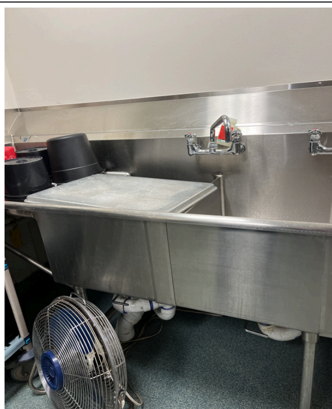
4/8/2024 - 221-4 - Nashua Elementary School- Kitchen - West Sink
