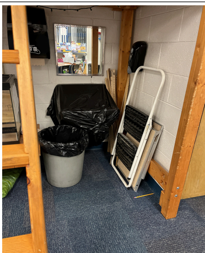
4/8/2024 - 221-28 - Nashua Elementary School- Room 11 - Handwashing Sink - Out of Order
