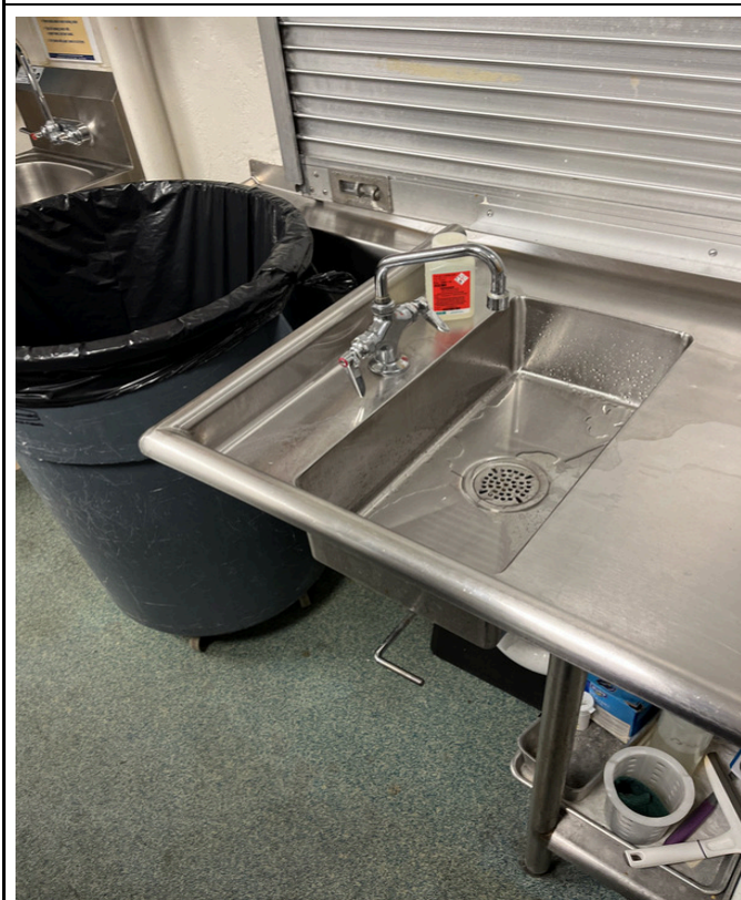
4/8/2024 - 221-3 - Nashua Elementary School- Kitchen - South Sink
