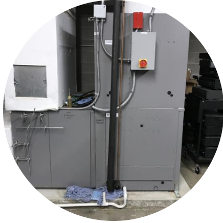
AHU Replacement + DDC Controls
