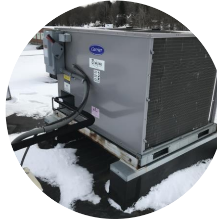
Condensing Unit Replacement
