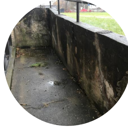
Repair & Replace Lightwells
