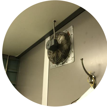
Exhaust Fans Replacement
