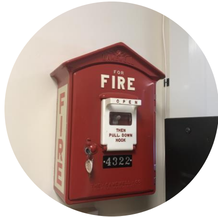
Replace Fire Alarm Systems
