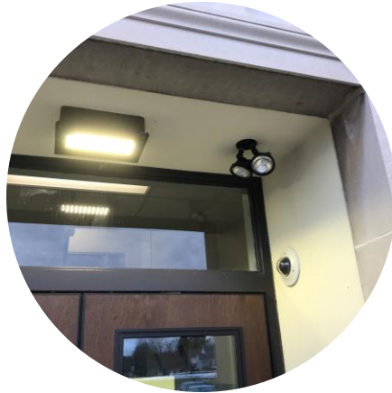
Replace Exterior Building Lighting
