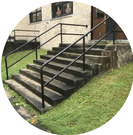
Exterior Stair @ Cafeteria
