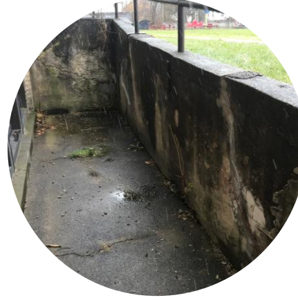
Repair & Replace Lightwells
