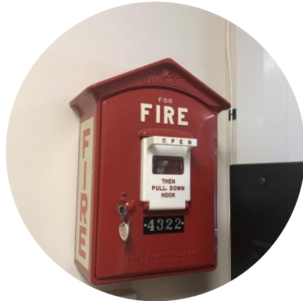
Replace Fire Alarm Systems
