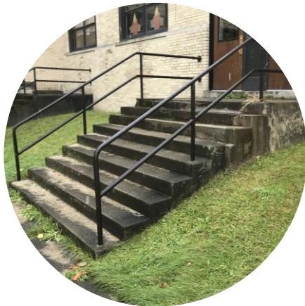
Exterior Stair @ Cafeteria
