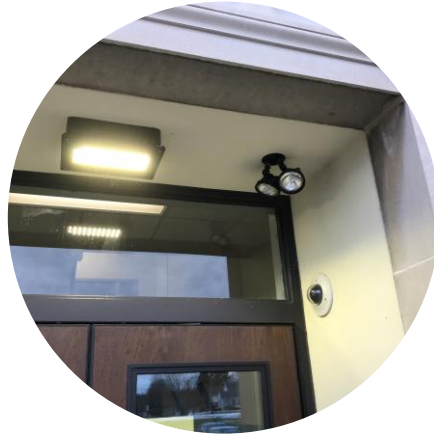
Replace Exterior Building Lighting
