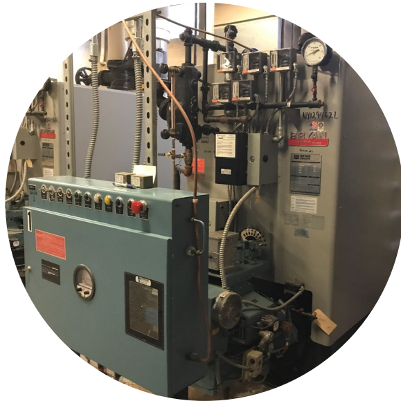
Replace End of Life Boilers
