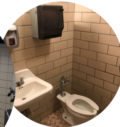
Staff & Student Bathroom Renovations
