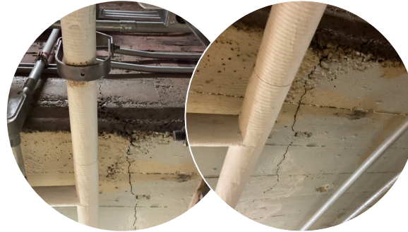
Repair Structural Cracks
