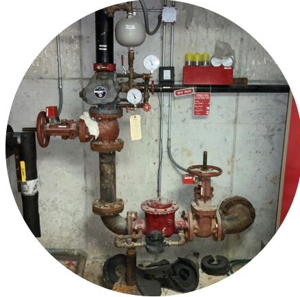
Replace Original, 70 Year Old Plumbing
