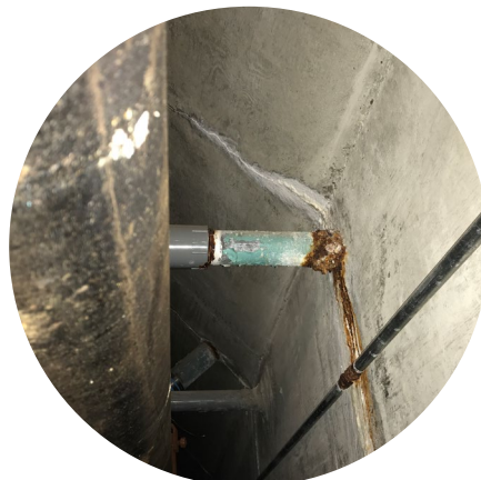
Replace Failing Pool Piping
