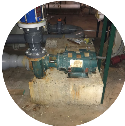
Replace Failing Pool Systems
