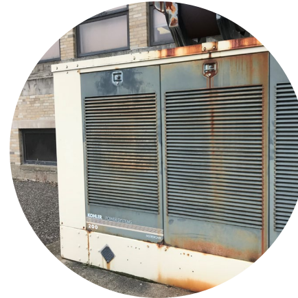
Replace Old Generator to Power Building Systems
