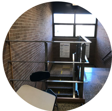
Replace Stair Railings for Student Safety
