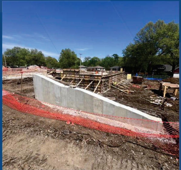
Admin Area Concrete Install
