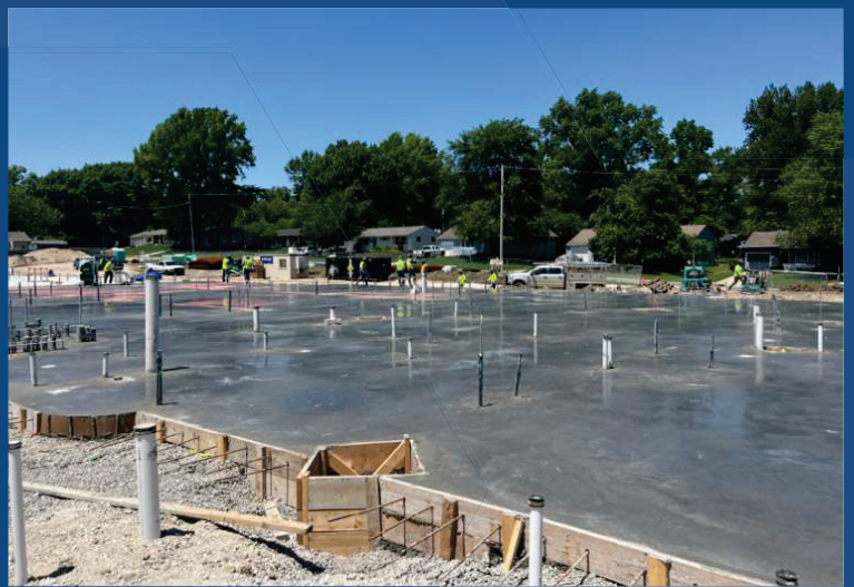
Area B North Slab Install
