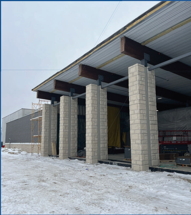
Exterior Masonry & Stone Install
