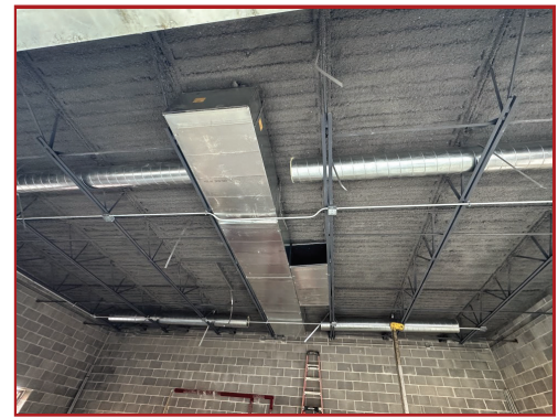
MEP Rough-In at Addition Ceiling
