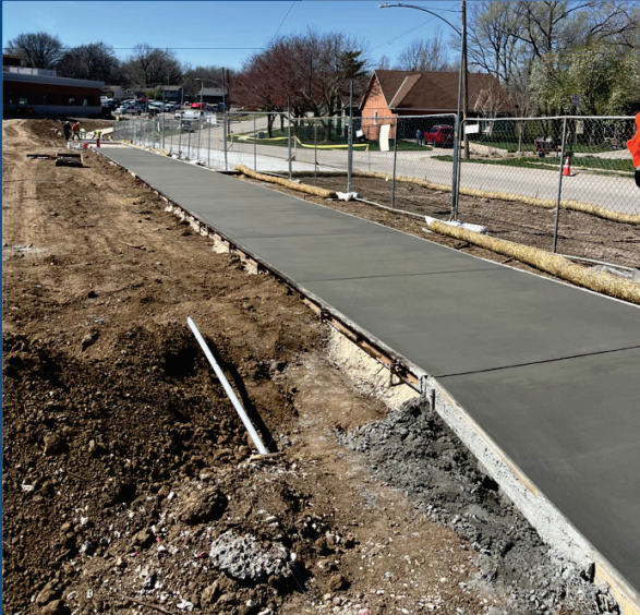
North Sidewalk Installation
