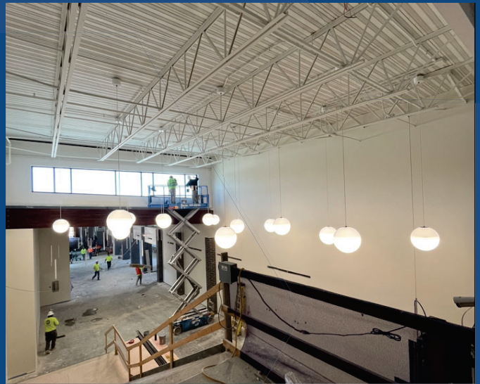
Area C Light Fixture Install
