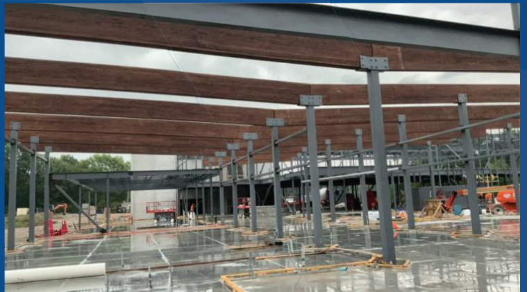
GluLam Beam Install
