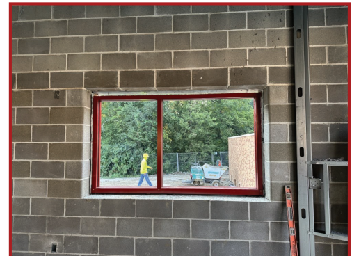
Addition Storefront Window Framing
