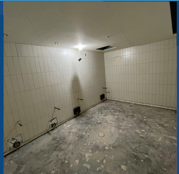
Area C Bathroom Tile Install
