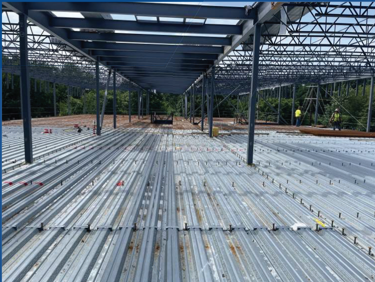
Area D Slab on Deck Preparation
