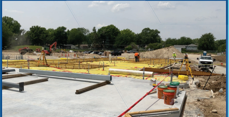
Area B Slab-on-Grade Prep.
