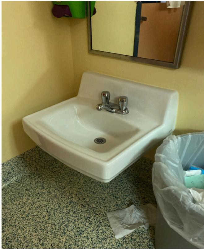
3/12/2024 - 9600-42 - ECC - 003799-Room 303- Unisex Restroom
