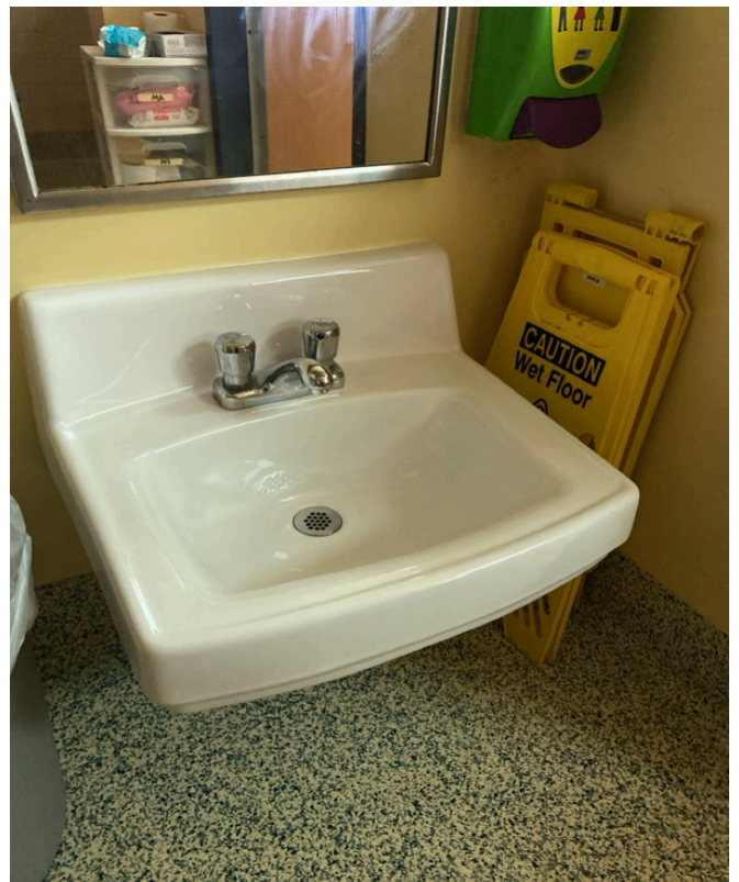
3/12/2024 - 9600-41 - ECC - 003798-Room 303 Unisex Restroom
