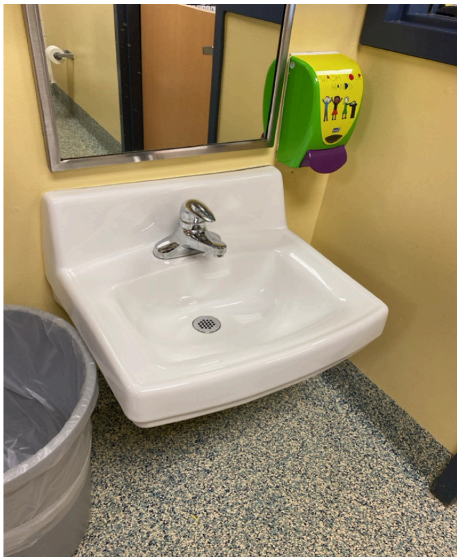
3/12/2024 - 9600-19 - ECC - 002030-Between 205-206-Right
