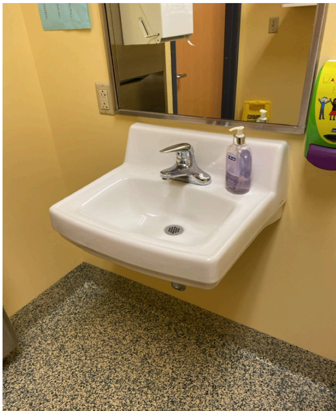
3/12/2024 - 9600-53 - ECC - 002011-Staff Restroom by 308
