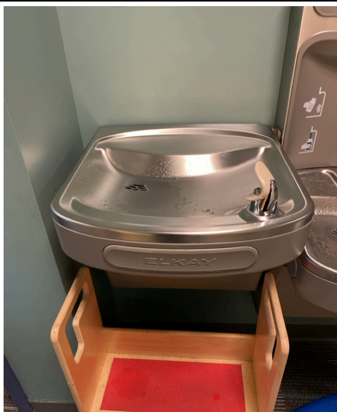
3/12/2024 - 9600-34 - ECC - 002045-Next to 204
