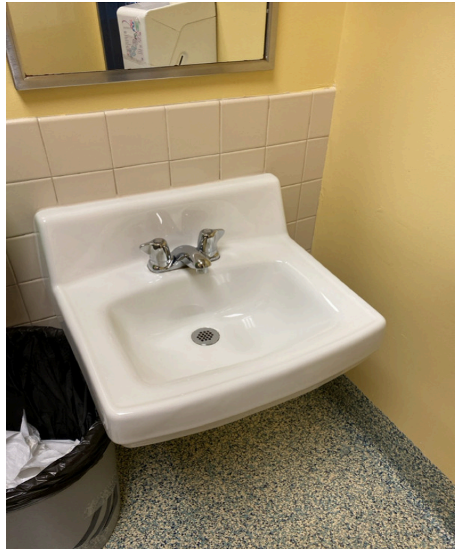
3/12/2024 - 9600-38 - ECC - 003794-Room 301- Unisex Restroom
