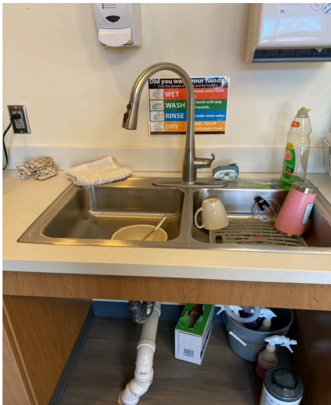
3/12/2024 - 9600-44 - ECC - 002002-Room 305- Lounge
