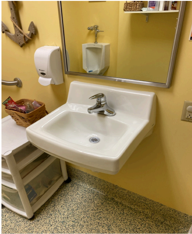
3/12/2024 - 9600-25 - ECC - 002036-Staff Restroom Across from 207
