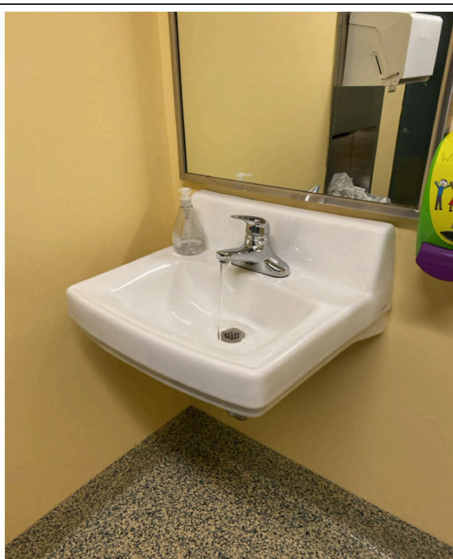
3/12/2024 - 9600-10 - ECC - 003790-Room 400-Staff Restroom
