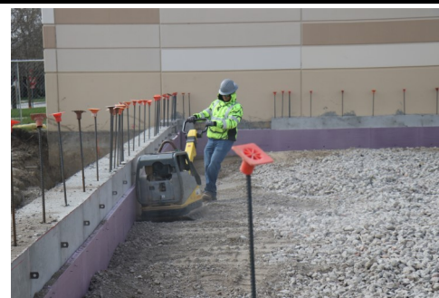
Field House Weight Room Construction
