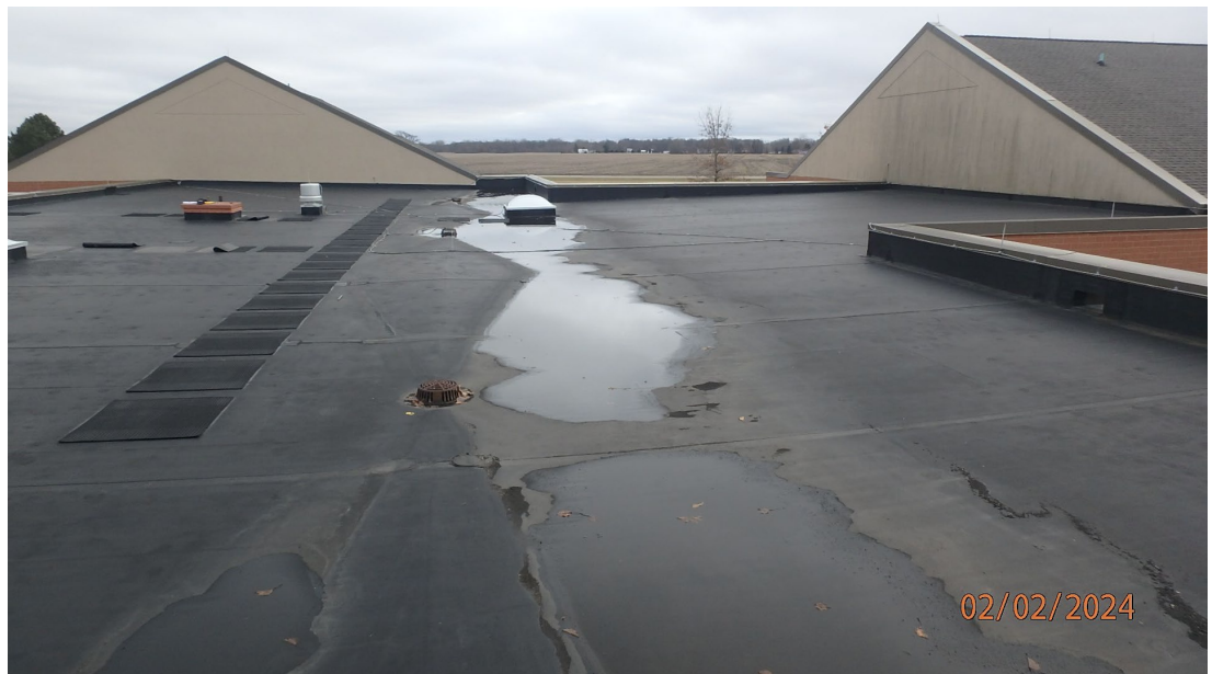
1.1.3.13 Overall view showing there is significant ponding along the drain line on Roof Area I. This will need to be corrected by the addition of tapered insulation around the roof drains, removing the existing crickets, and installing new properly located crickets.
