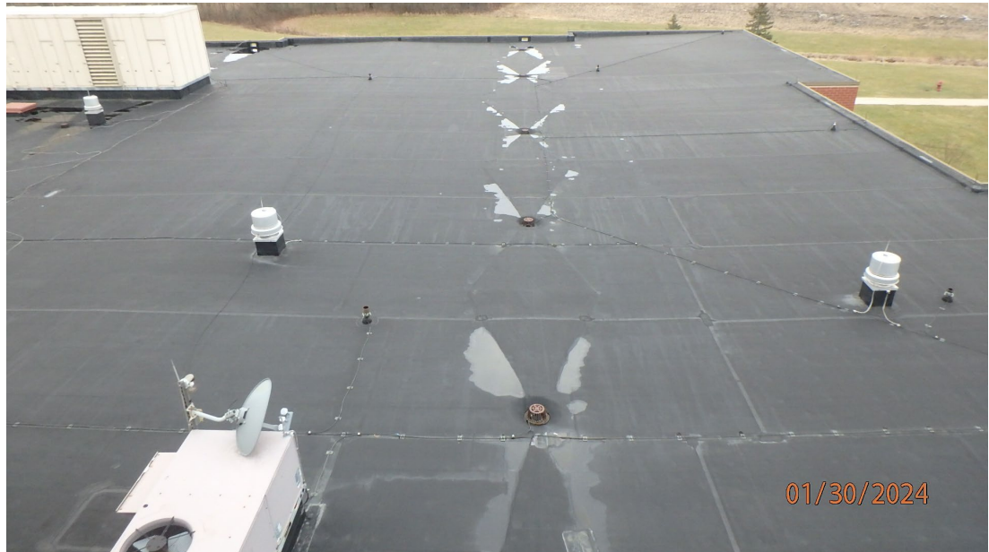
1.1.2.4 View of a line of roof drains on Roof Area D showing there is no significant ponding water. There is some minor ponding water near the roof drains. This can be corrected with addition of tapered insulation around the roof drains.
