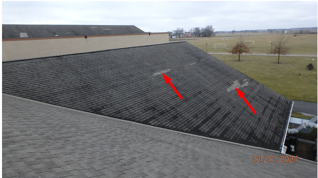
1.1.4.3 Overall view of Roof Area B3 where there has been shingle replacement due to shingles blowing off during high winds.
