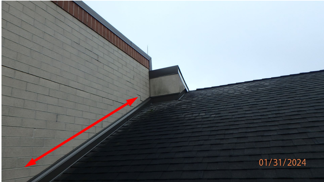
1.3.20 River Valley High School – View of an area where there is no apparent through wall flashing above the steep sloped roof area.
