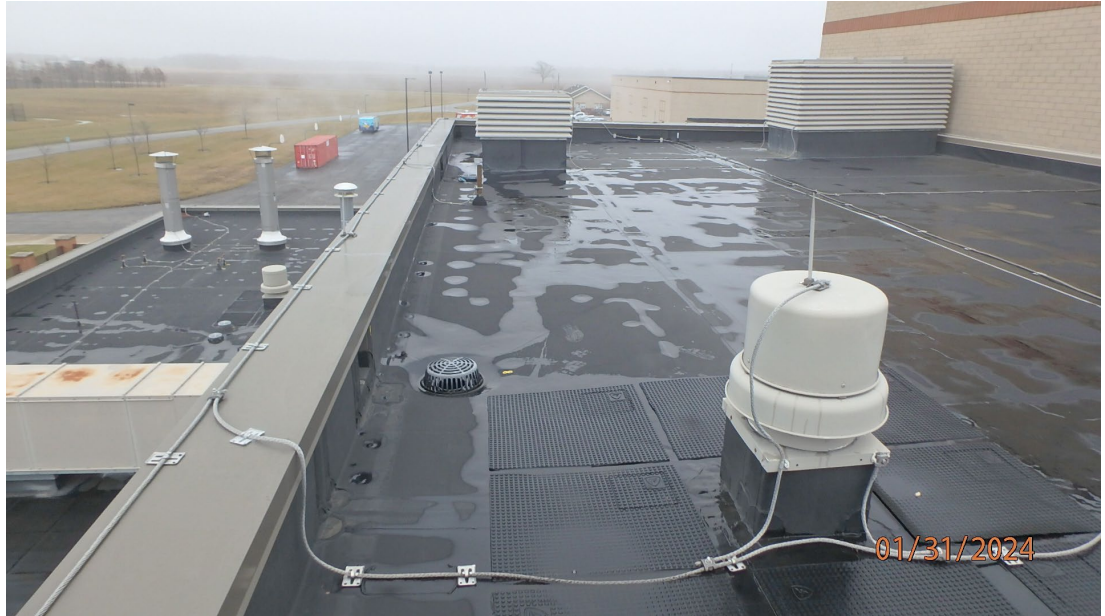
1.1.4.13 View of an area on Roof Area O showing there is no significant ponding on this roof area.
