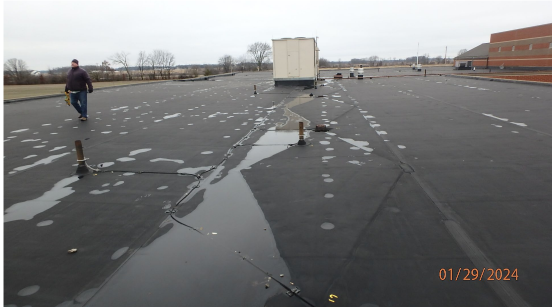
1.1.1.6 Close-up view of the same area from the previous photograph showing that there is some ponding water along this drain line. Tapered insulation around the roof drains and tapered insulation crickets can be installed to improve the drainage at this area.
