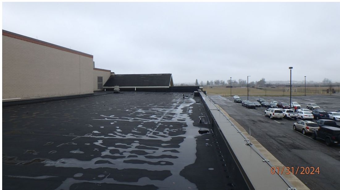
1.1.4.10 View of an area on Roof Area N showing there is no significant ponding on this roof area. Additional tapered insulation would be installed around the drains and larger crickets installed between the roof drains to improve the drainage.
