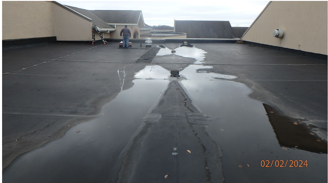
1.1.3.8 Overall view showing there is significant ponding along the drain line on Roof Area C. This will need to be corrected by the addition of tapered insulation around the roof drains and possibly larger tapered insulation crickets.
