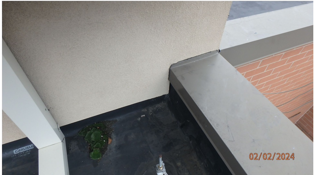
1.3.5.2 River Valley Middle School – View of an area where the EIFS will need to be modified so that a watertight transition can be provided at the coping cap. In addition, the base flashing height may need to be raised to accommodate the new roof system.
