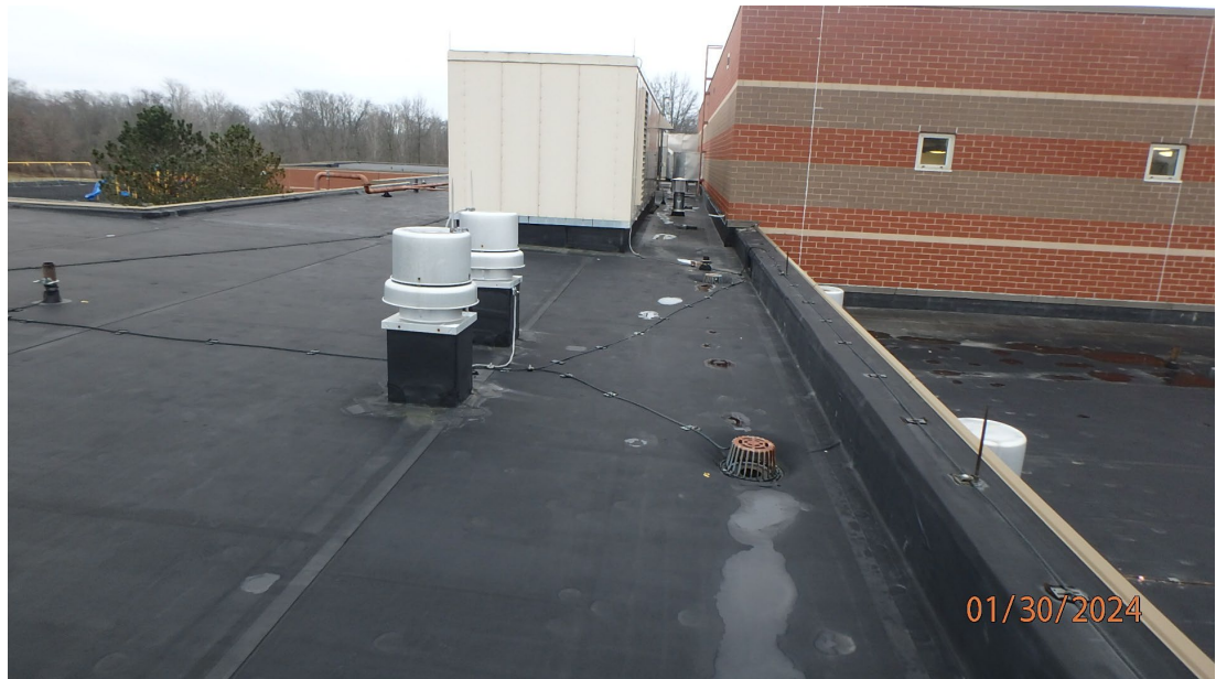
1.1.2.1 View of a line of roof drains on Roof Area A showing there is no significant ponding water.
