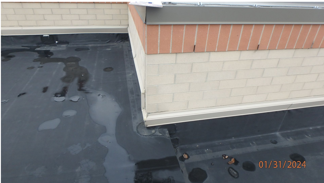
1.3.23 River Valley High School – View of an area where there are no weeps observed above the receiver.
