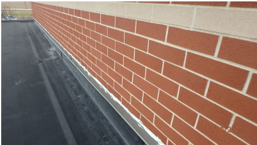
1.3.7 Liberty Elementary - View of an area where asphalt can be seen extending out from under the brick veneer at the sheet metal flashing.
