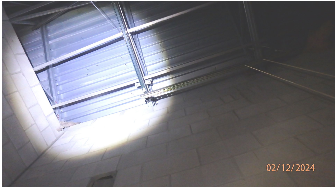
1.4.2.4 View above the drop ceiling at an adjacent hallway area, where a frozen sprinkler line/head was reported. There is no drywall attached to the bottom of the cold-formed metal trusses at these locations and there is no air barrier between the top of the wall and the bottom of the roof deck.
