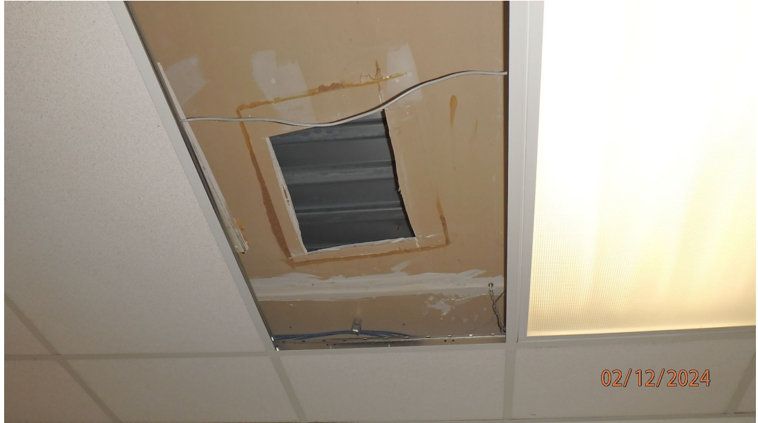
1.4.1.1 View of the construction above the drop ceiling at a classroom area. Drywall has been installed across the bottom of the cold-formed metal trusses. We removed a previously installed cover panel to see the eave detail.
