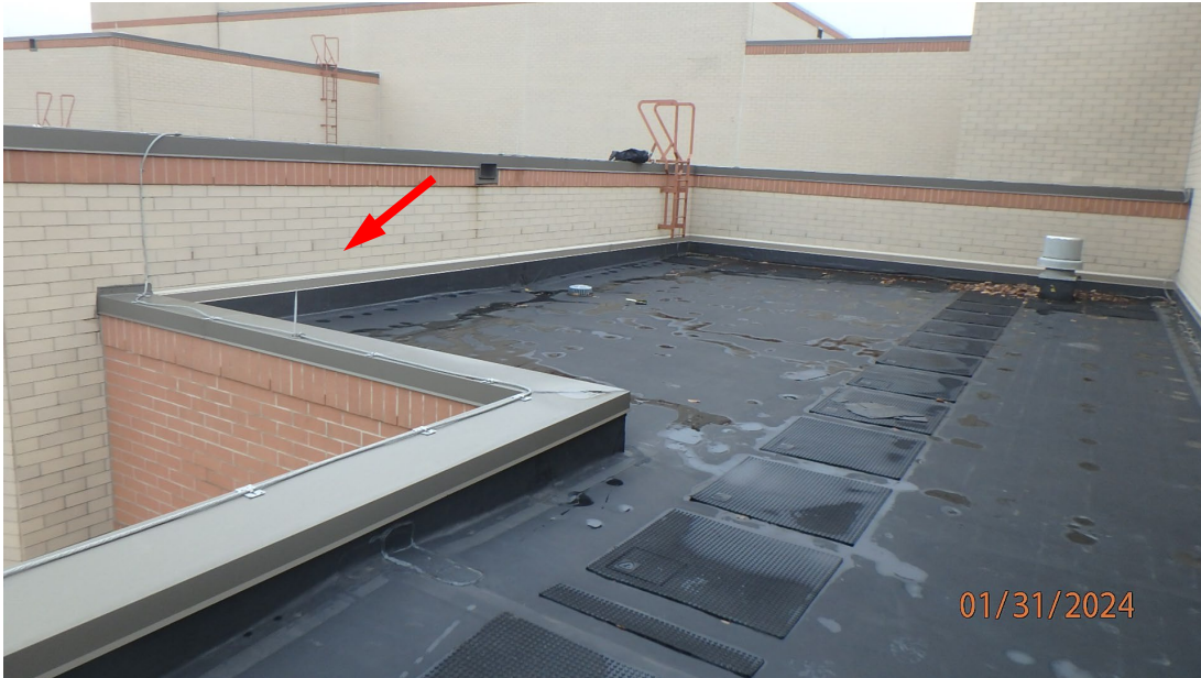
1.3.22 River Valley High School – Overall view of an area where the weeps are 3 courses above the receiver.
