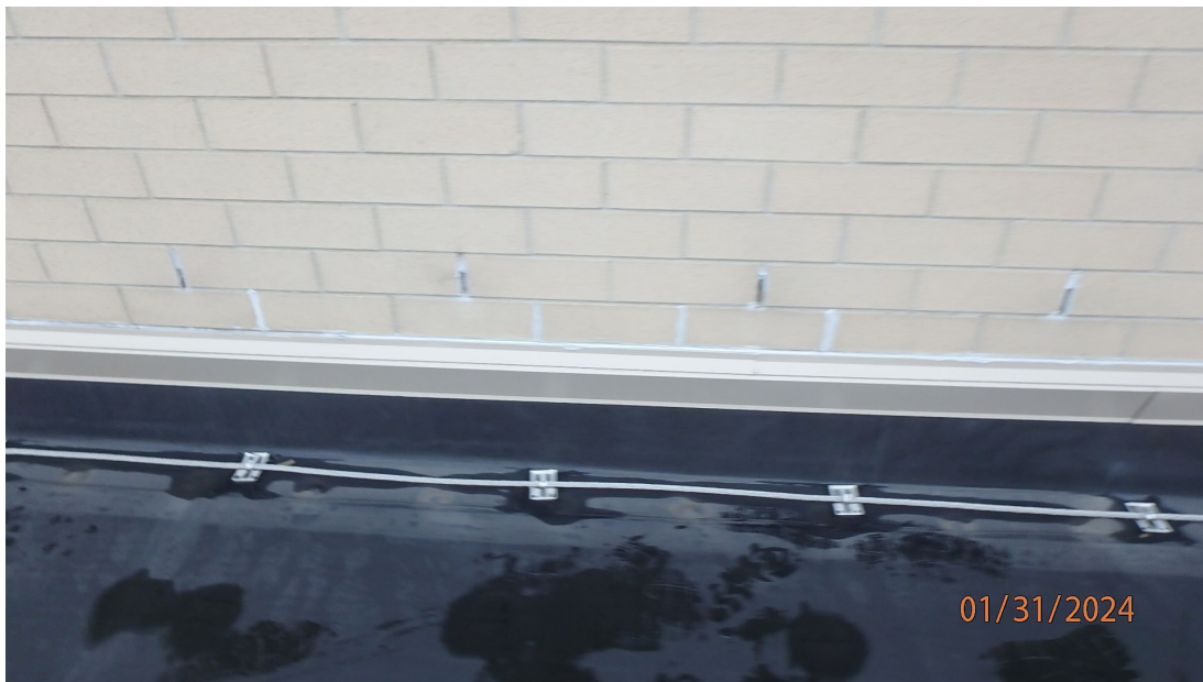
1.3.17 River Valley High School – View of an area where the weeps are one (1) course above the receiver.
