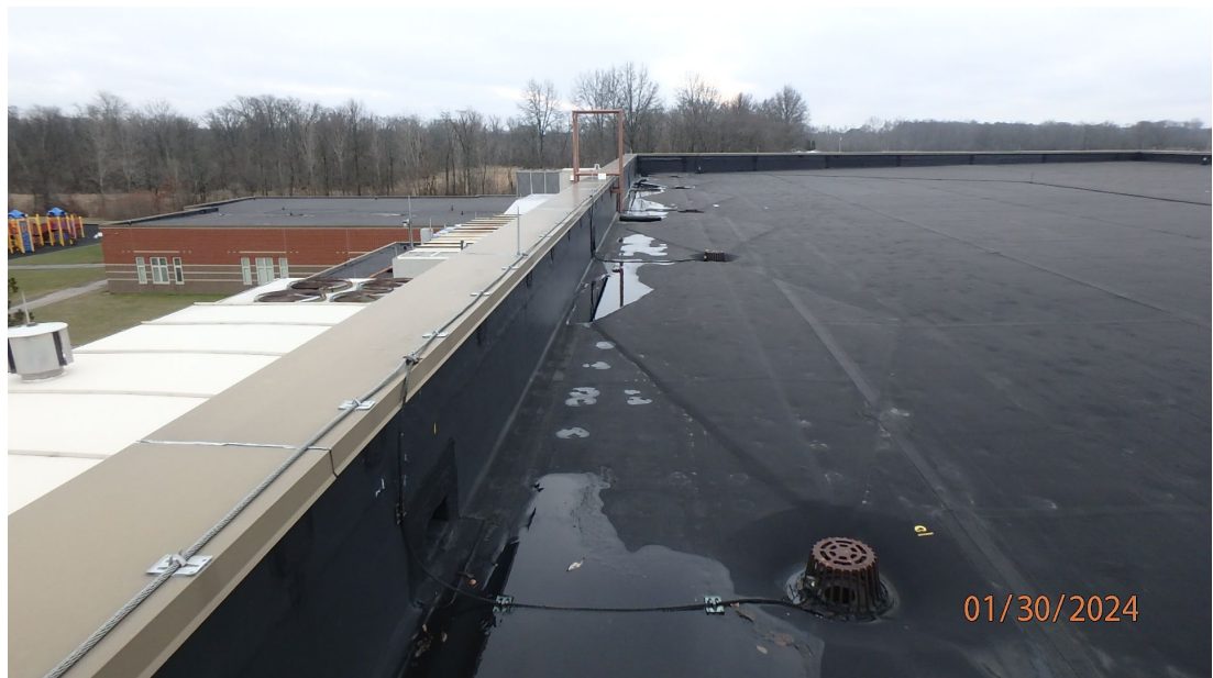
1.1.2.3 View of a line of roof drains on Roof Area C showing there is no significant ponding water. There is some minor ponding water near the roof drains. This can be corrected with addition of tapered insulation to create back slope to the roof drains and tapered insulation around the roof drains.
