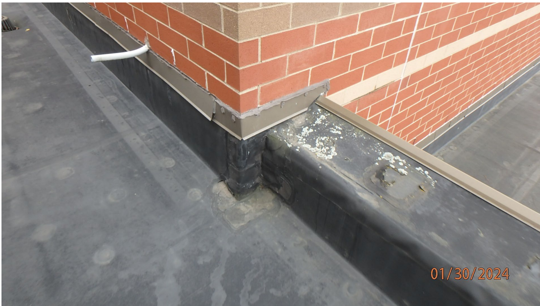
1.3.5 Liberty Elementary - View showing a sheet metal flashing has been installed at the masonry through wall flashing location, but it is not a 2-piece flashing that allows it to be removed to replace the roof base flashing.
