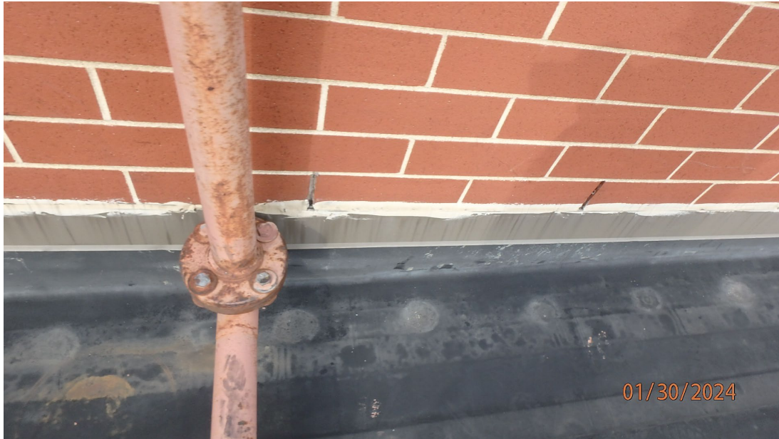
1.3.6 Liberty Elementary - View of an area where additional sealant has been installed between the sheet metal flashing and brick masonry.
