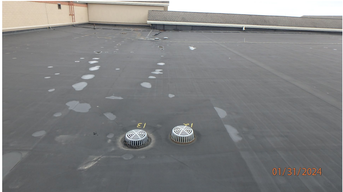
1.1.4.9 View of an area on Roof Area N showing there is no significant ponding on this roof area.
