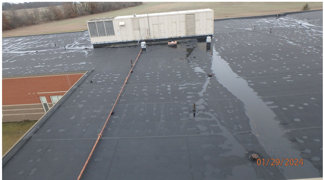
1.1.1.7 Another overall view of Roof Area D. There is ponding along this line of roof drains that can be addressed during the roof replacement by adding tapered insulation around the roof drains and adding larger tapered insulation crickets.
