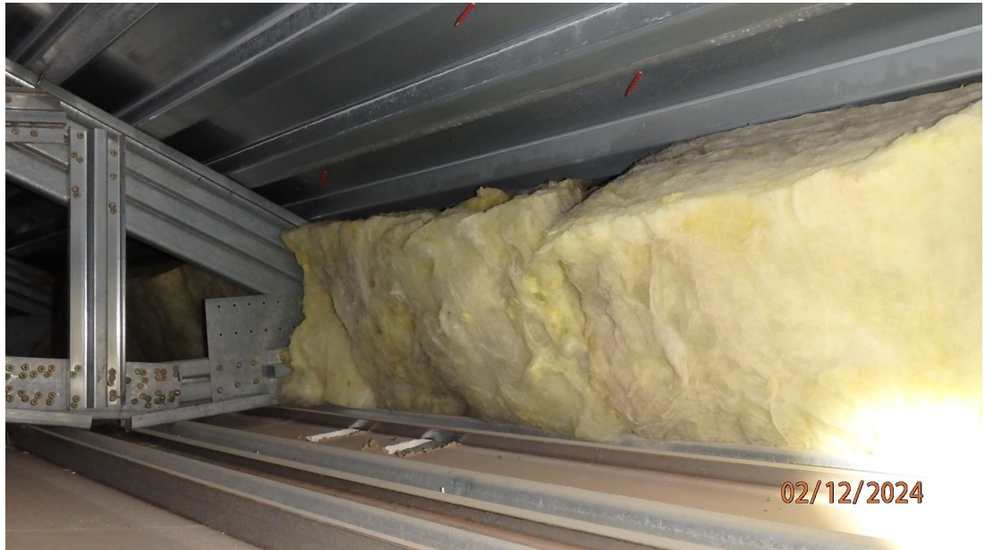
1.4.1.2 View showing batt insulation has been installed between the roof deck and the top of the wall.
