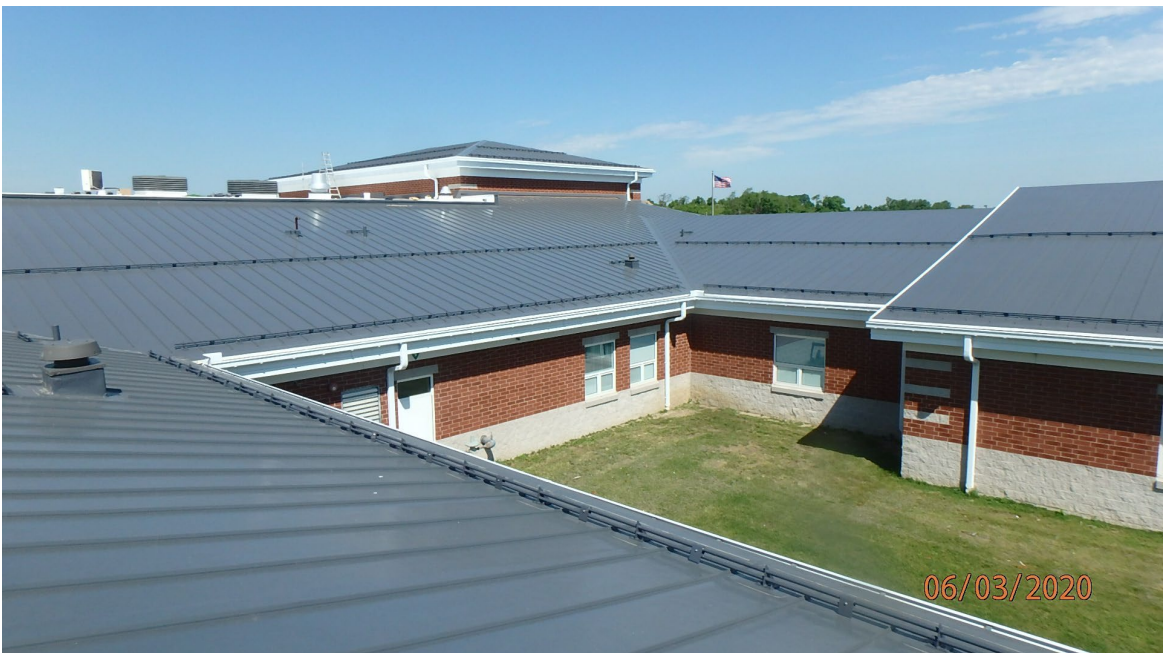
1.2.2.4 Overall view of a typical colored thermoplastic membrane roof system with aesthetic ribs.
