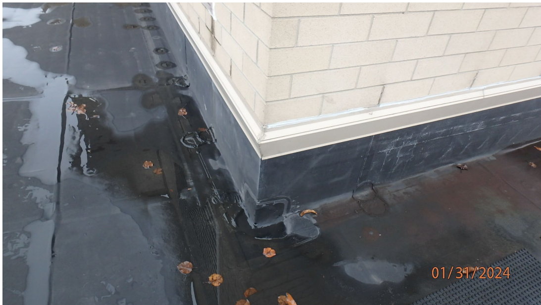
1.3.15 River Valley High School – Close-up view showing a 2-piece counterflashing has been installed at the through wall flashing location. Sealant has been installed between the sheet metal receiver and brick masonry.
