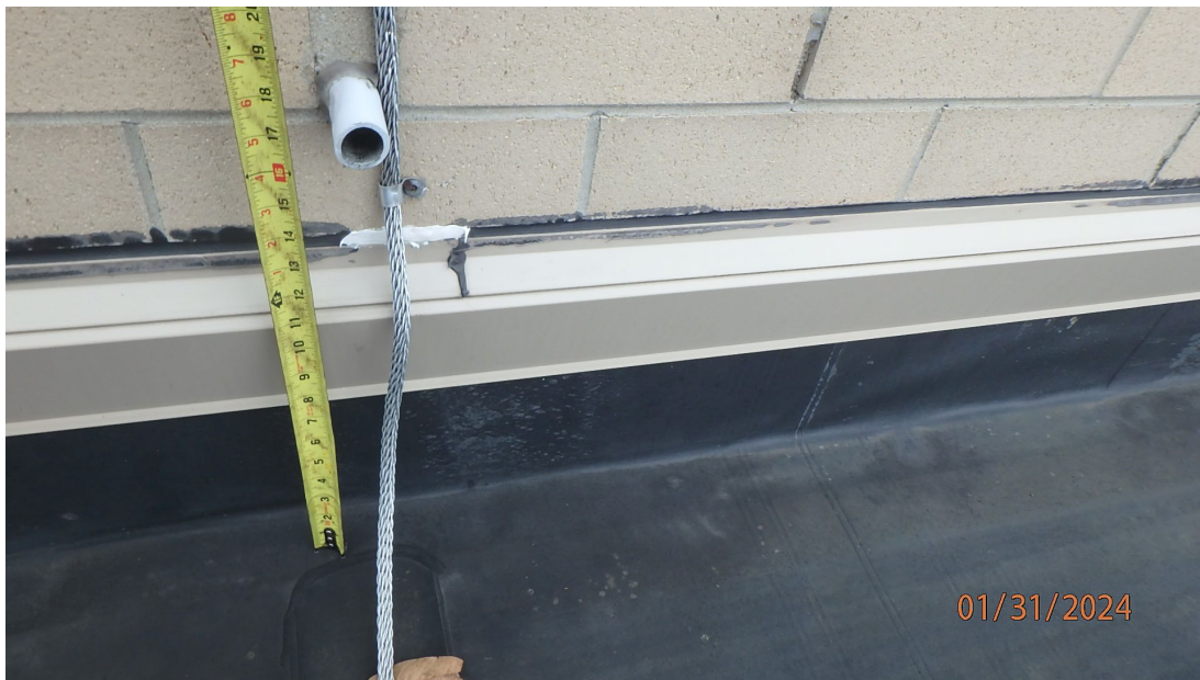
1.3.21 River Valley High School – Close-up view of an area where the weeps are installed 1 course above the receiver and sealant has been installed between the receiver and the brick masonry.
