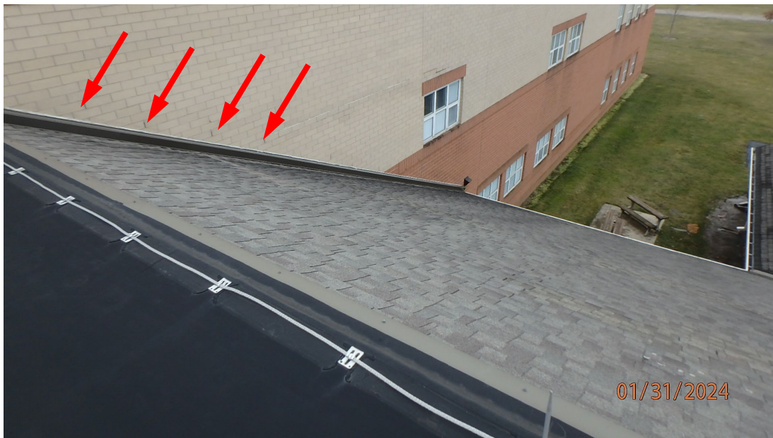
1.3.25 River Valley High School – View of a steep sloped roof area where there are weeps above the roof, but there are no stepped counterflashings installed to eliminate unflashed masonry.
