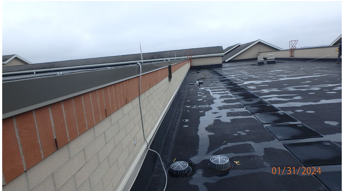
1.1.4.5 View of an area on Roof Area D2 showing there is no significant ponding on this roof area.
