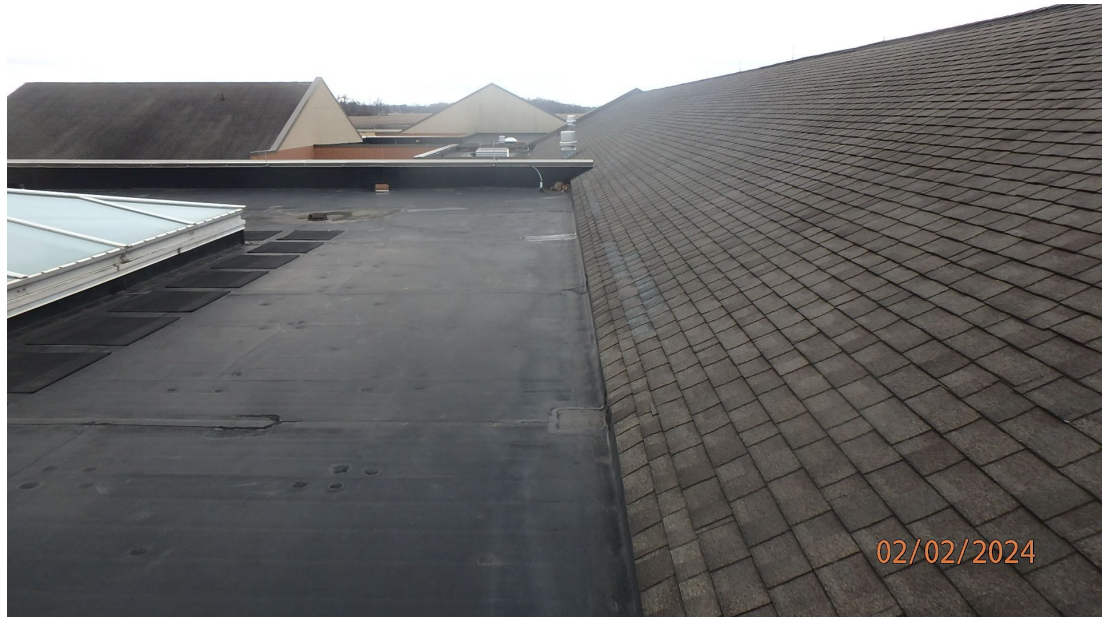
1.1.3.7 View along this tie-in area showing steep slope roof extends beyond Roof Area B.
