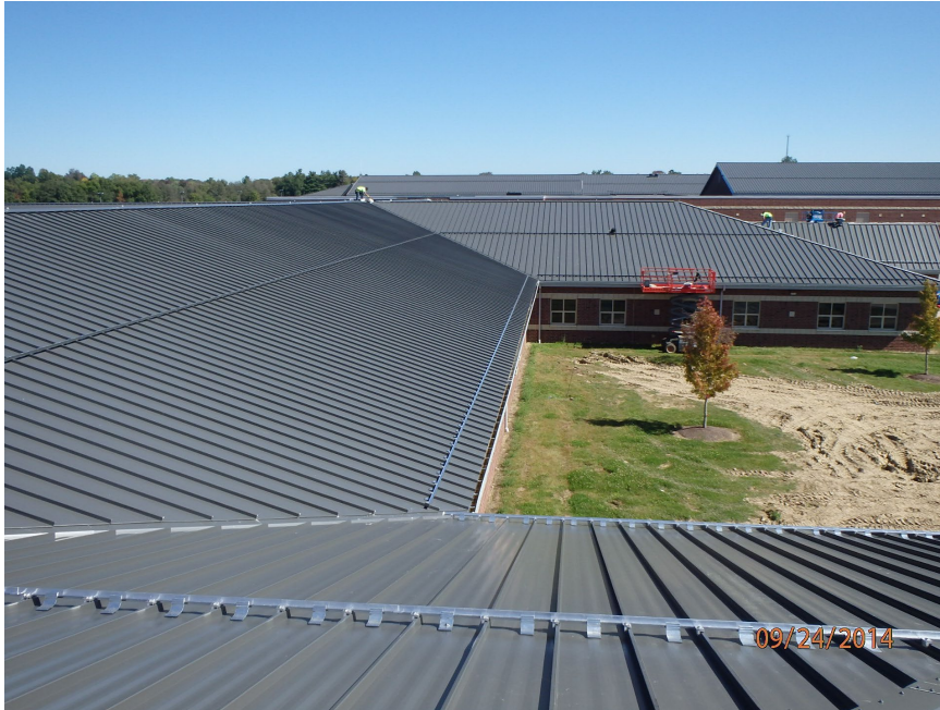
1.2.2.1 Overall view of a typical standing seam metal roof system.
