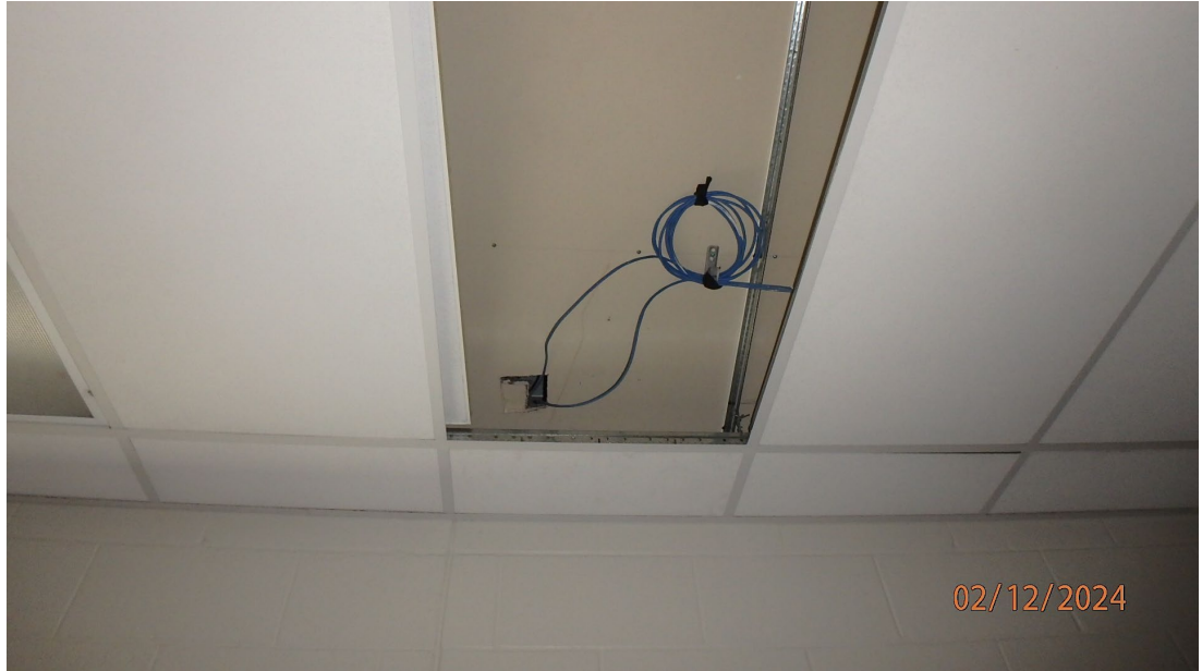
1.4.2.1 View of the construction above the drop ceiling at a classroom area. Drywall has been installed across the bottom of the cold-formed metal trusses.
