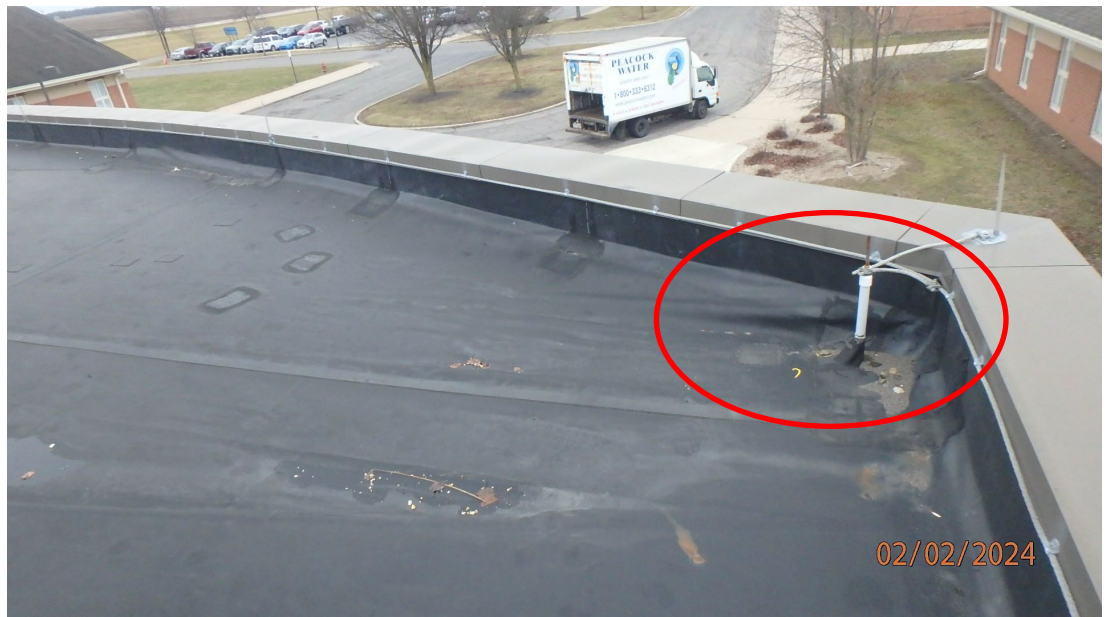
1.1.3.11 View of an area on Roof Area F where the roof membrane shrinkage is starting to pull the roof membrane off of the wall. This type of failure starts to occur as the roof membrane ages.
