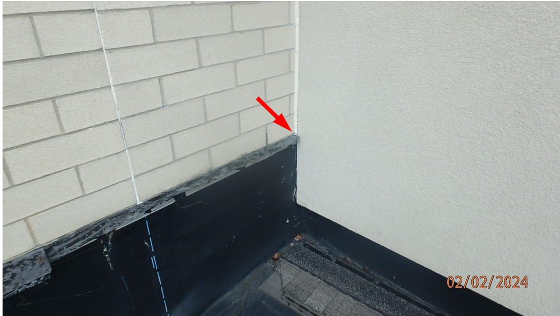
1.3.12 River Valley Middle School – View of a masonry through wall flashing that is terminated in the middle of a brick, so it cannot be properly end dammed.
