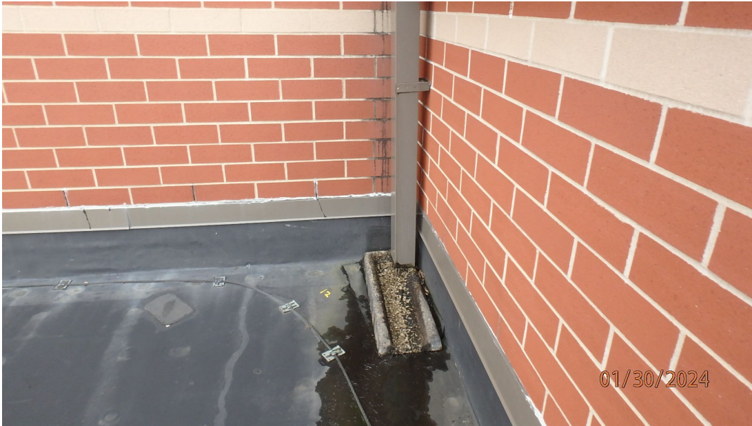
1.3.4 Liberty Elementary - View showing a sheet metal flashing has been installed at the masonry through wall flashing location, but it is not a 2-piece flashing that allows it to be removed to replace the roof base flashing.
