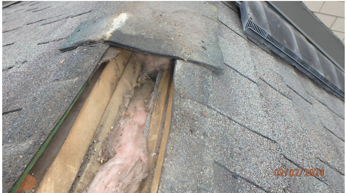
1.1.3.2 View showing fiberglass batt insulation has been installed between the rigid insulation, which was not continuous at the ridge.
