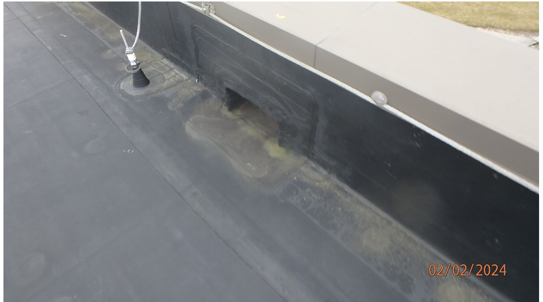
1.3.3.2 River Valley Middle School – View of a roof overflow drainage scupper that will need to be modified to accommodate the new roof system.
