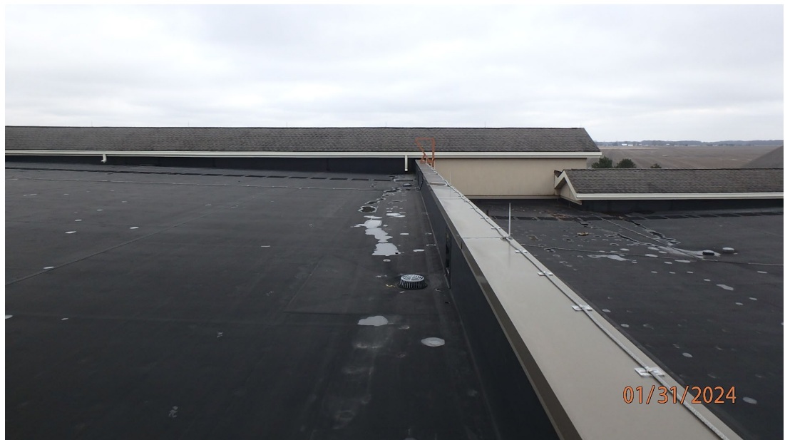
1.1.4.8 View of an area on Roof Area L showing there is no significant ponding on this roof area.
