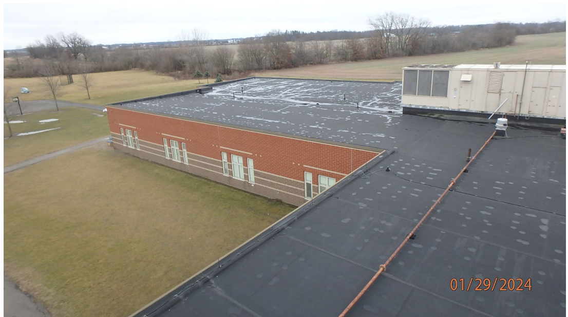
1.1.1.5 Overall view of roof area D showing there is no significant ponding water.
