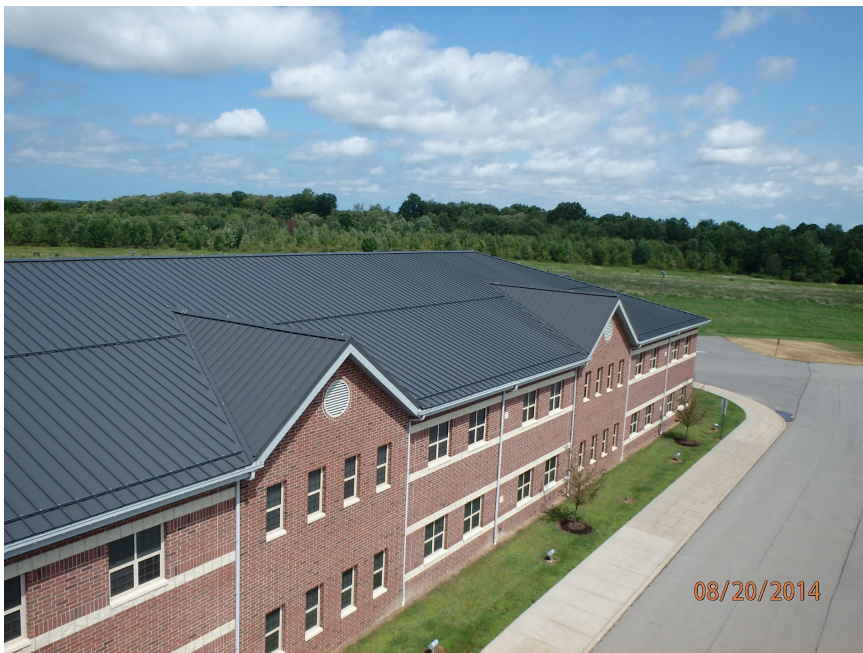
1.2.2.2 Overall view of a typical standing seam metal roof system.
