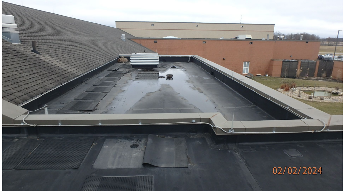
1.1.3.12 Overall view showing there is significant ponding along the drain line on Roof Area G. This will need to be corrected by the addition of tapered insulation around the roof drains and possibly larger tapered insulation crickets.
