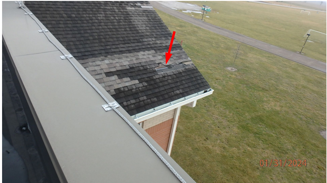
1.1.4.7 Overall view of Roof Area F1 where there has been shingle replacement due to shingles blowing off during high winds. There are currently additional shingles that have blown off and need to be replaced.
