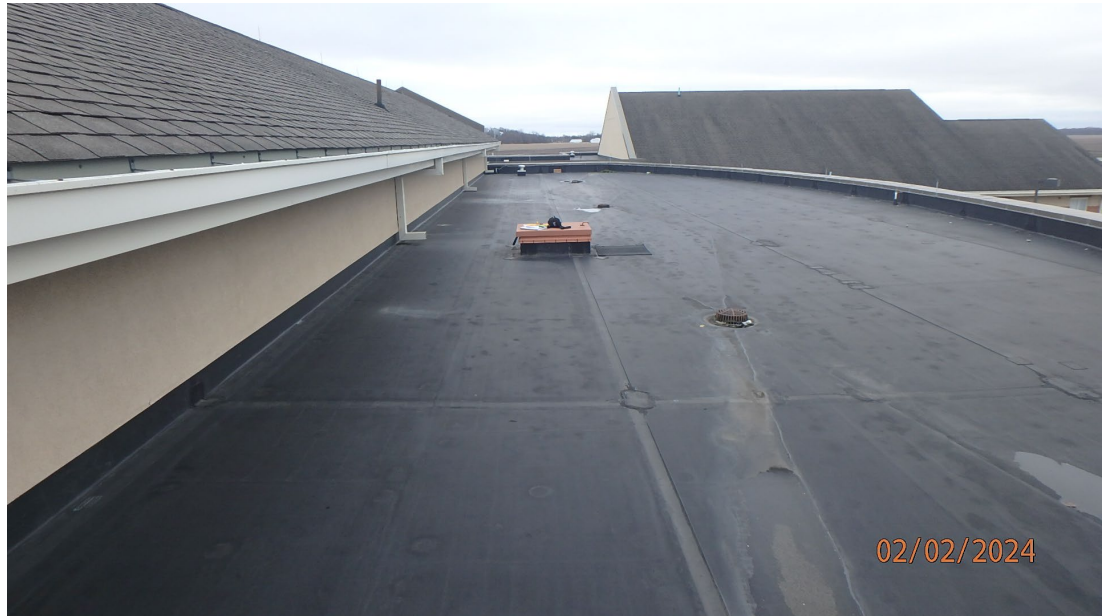
1.1.3.10 View of an area on Roof Area F showing there is no significant ponding on this roof area.
