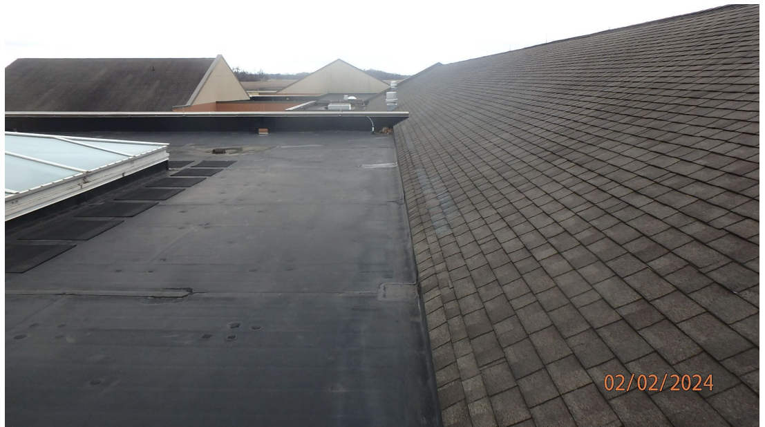
1.3.2.1 River Valley Middle School – View of an area where the steep slope roof directly ties into the low-sloped roof system.
