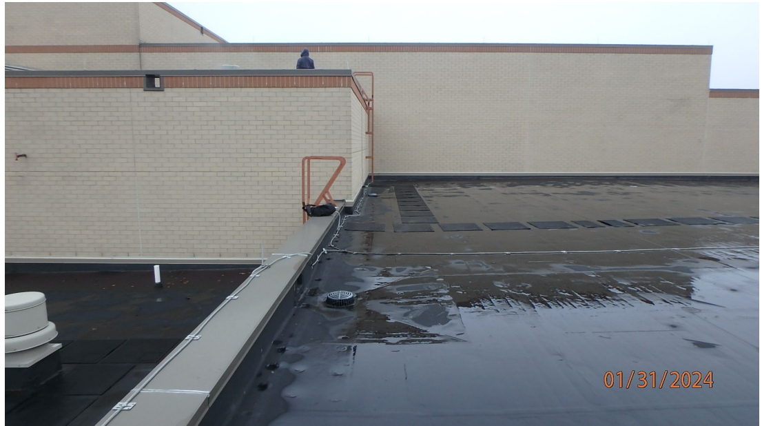
1.1.4.11 View of an area on Roof Area N showing there is no significant ponding on this roof area.
