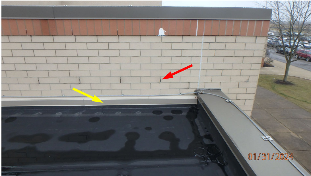
1.3.14 River Valley High School – View of an area where the weeps (red arrow) are 2 courses higher than the counterflashing (yellow arrow), leaving 2 courses of masonry that are not flashed.
