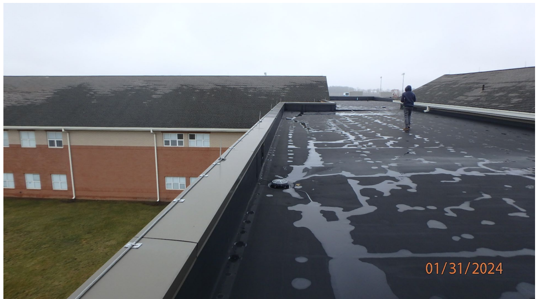
1.1.4.6 View of an area on Roof Area E showing there is no significant ponding on this roof area. Additional tapered insulation would be installed around the drains and larger crickets installed between the roof drains to improve the drainage.
