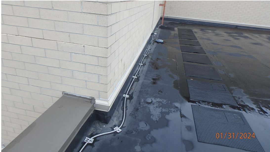
1.3.16 River Valley High School – View of another location where the masonry through wall flashing is not stepped up over the coping cap.
