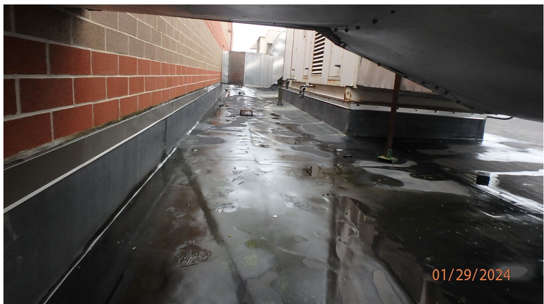
1.1.1.1 Overall view of Roof Area A, along a line of roof drains showing there is no significant ponding water at this area.
