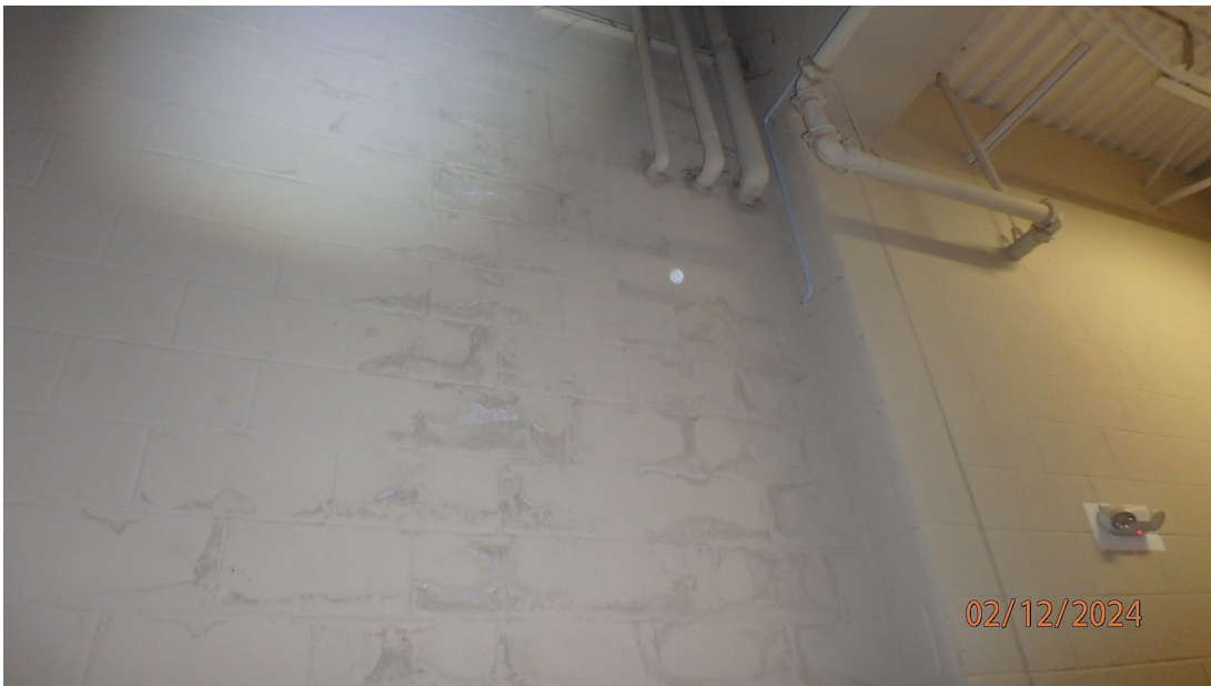
1.3.19 River Valley High School – View of an area at the rear of the stage where there is efflorescence in the masonry wall. Efflorescence is caused by moisture and this damage could be related to leakage at the masonry through wall flashing.
