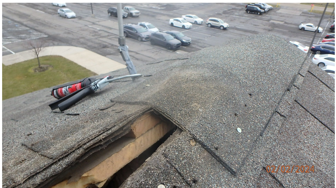
1.1.4.2 View showing that the rigid insulation was not tightly mitered together and there was no fiberglass batt insulation installed between the rigid insulation at the ridge on this building. There was a gap between the rigid insulation of approximately 6" at this location.
