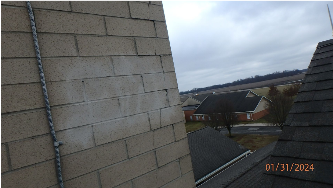
1.3.26 River Valley High School – View of crack observed in the masonry at an outside corner.
