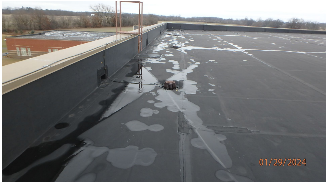
1.1.1.4 Overall view of Roof Area C showing there is no significant ponding water. There is some minor ponding water near the roof drains. This can be corrected with addition of tapered insulation around the roof drains.
