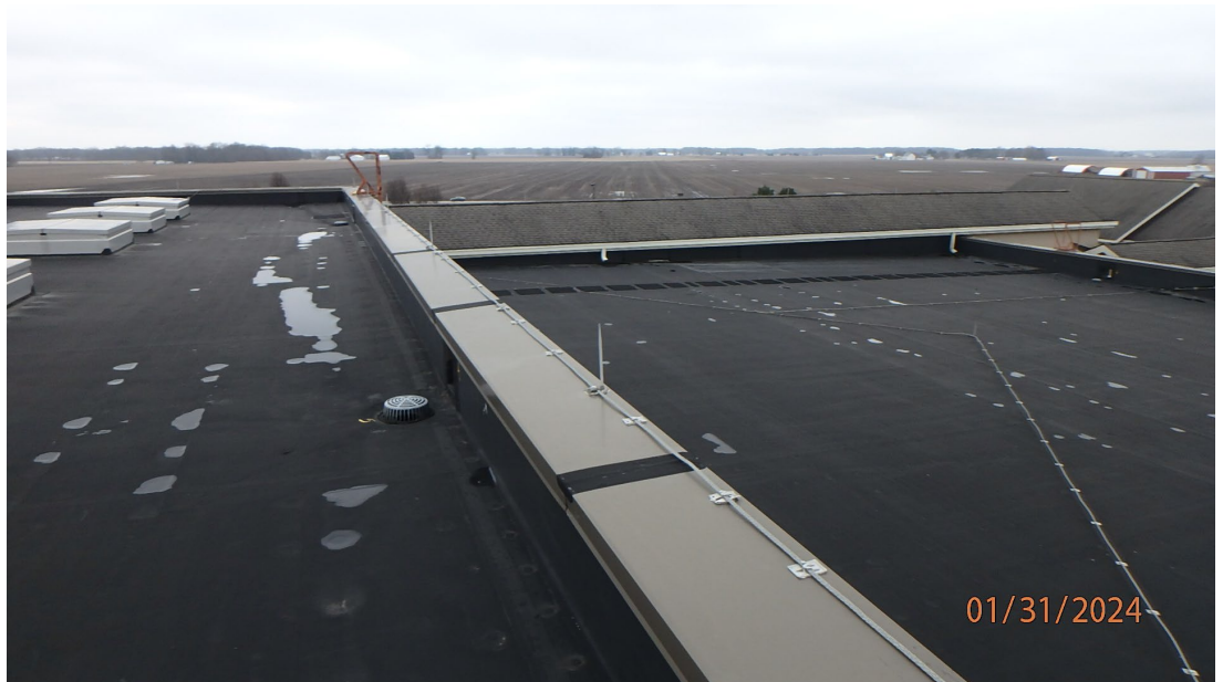
1.1.4.14 View of an area on Roof Area P showing there is no significant ponding on this roof area.
