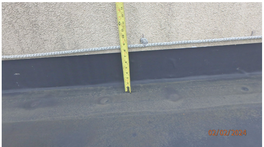
1.3.5.3 River Valley Middle School – View of an area where the EIFS will need to be modified in order to accommodate the height of the new roof system.
