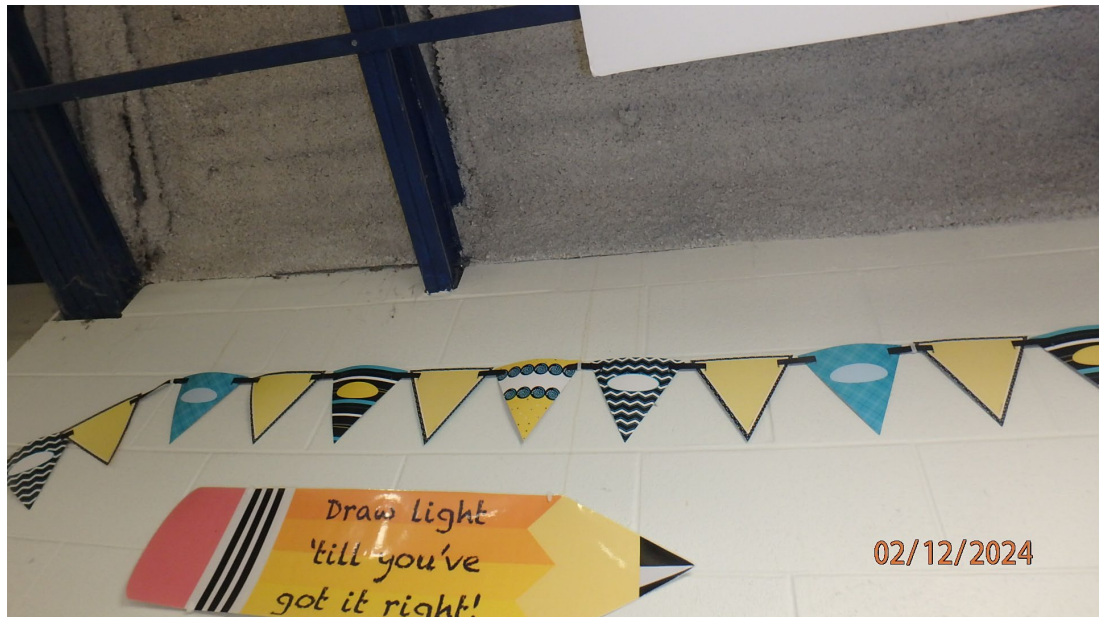
1.3.6.1 River Valley High School - View of the K-13 insulation installed on the bottom of the roof deck in Room 100.
