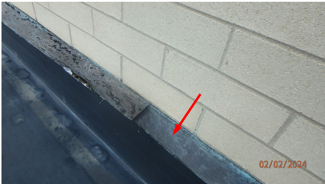
1.3.9 River Valley Middle School – Close-up view of the laminated copper masonry through wall flashing material.
