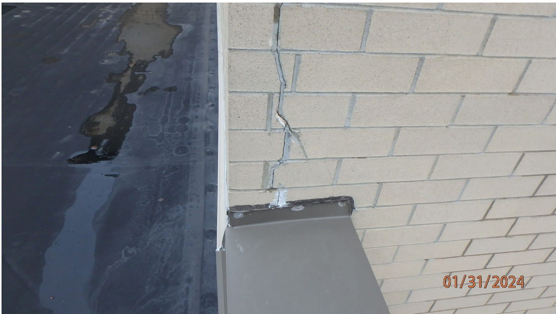
1.3.27 River Valley High School – View of crack in the masonry at another outside corner location.
