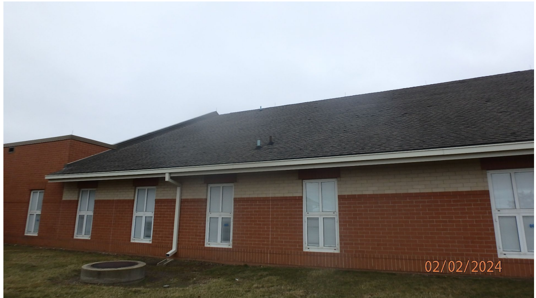
1.1.3.14 Overall view of Roof Area H2 there are numerous raised shingles on this roof area.
