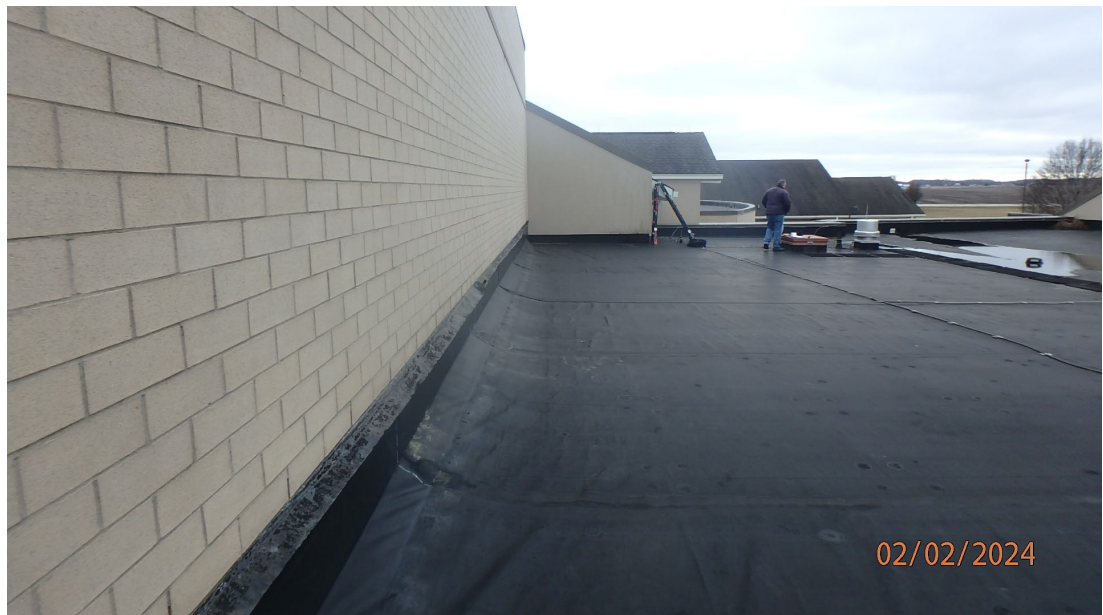
1.1.3.9 View of an area on Roof Area C where the roof membrane perimeter securement has been compromised and the roof membrane has started to become unadhered. This area should have some temporary securement installed to prevent further (and possibly severe) wind damage prior to the roof replacement being implemented.
