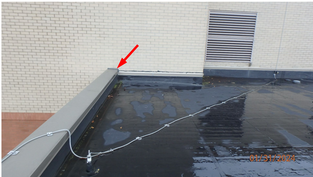
1.3.13 River Valley High School – View of an area where the masonry through wall flashing does not step up over the coping cap.
