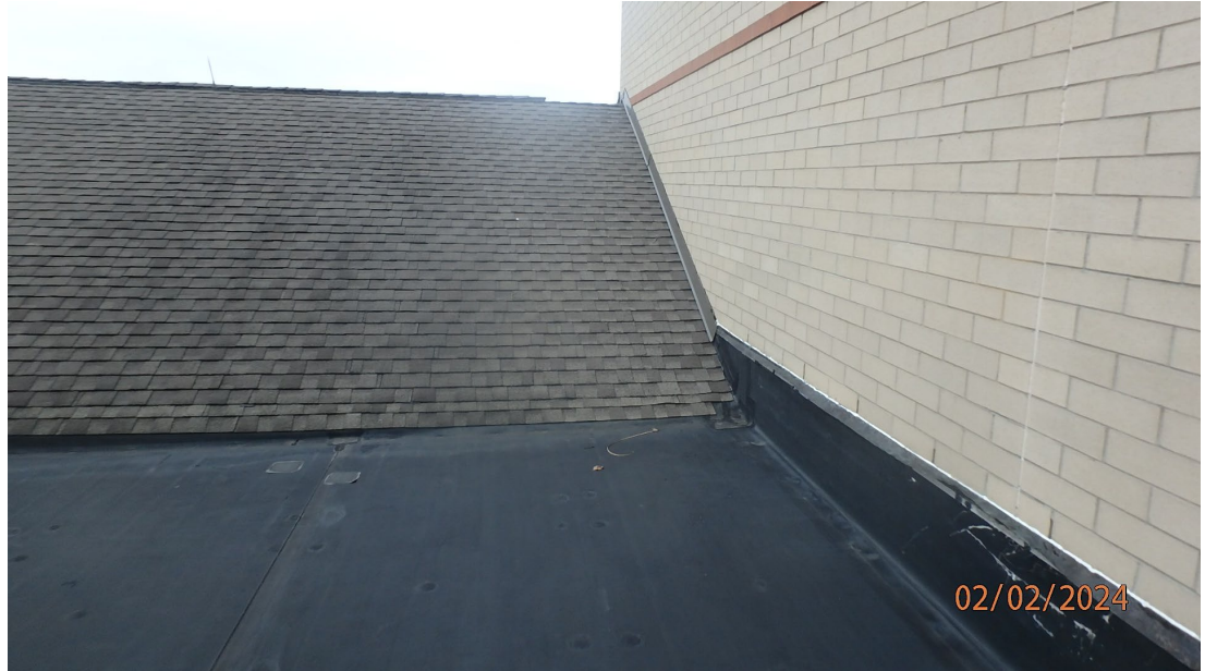
1.1.3.6 Overall view showing that a portion of Roof Area E1 (steep sloped shingle area) ties directly into Roof Area B (low sloped EPDM roof area).
