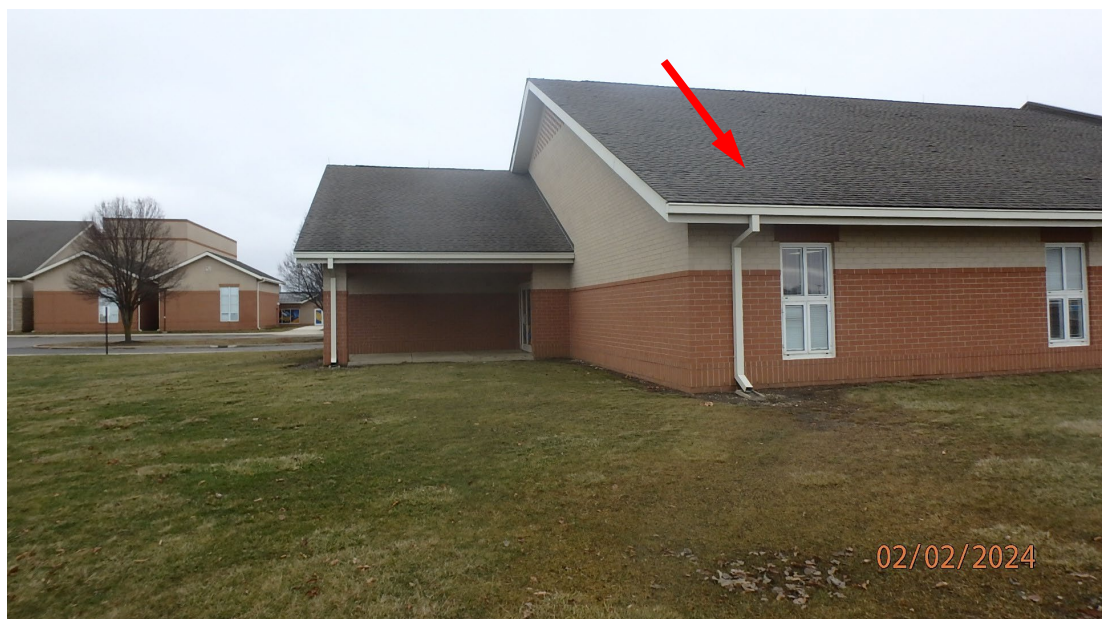
1.1.3.15 Overall view of Roof Area J2 there are numerous raised shingles on this roof area.
