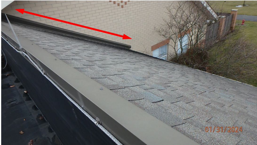
1.3.24 River Valley High School – View of another area where there is no apparent masonry through wall flashing above the steep sloped roof area.
