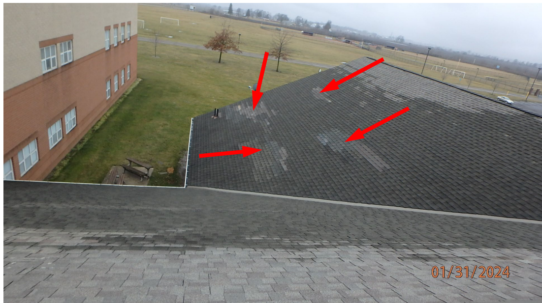
1.1.4.4 Overall view of Roof Area B4 where there has been significant shingle replacement due to shingles blowing off during high winds.
