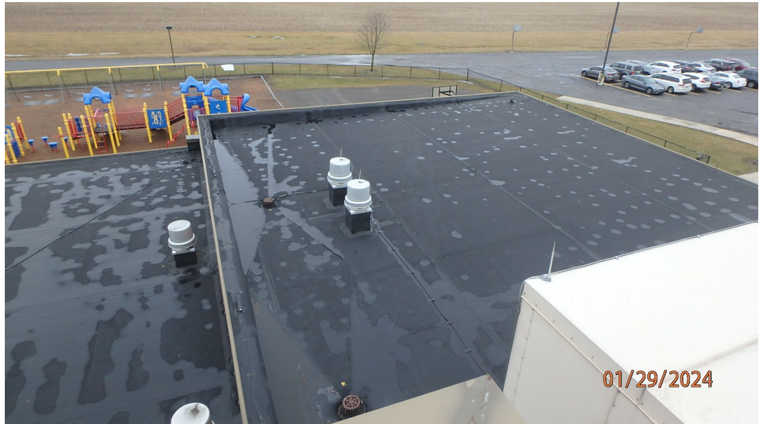
1.1.1.2 Overall view of Roof Area A, where tapered insulation is needed to create back slope and improve the roof drainage on this area.
