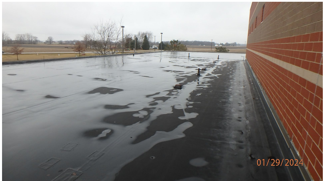
1.1.1.3 Overall view of Roof Area B showing there is no significant ponding water.
