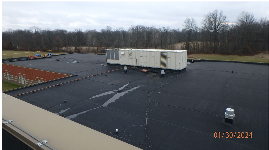
1.1.2.5 View of a line of roof drains on Roof Area D showing there is no significant ponding water. There is some minor ponding water near the roof drains. This can be corrected with addition of tapered insulation around the roof drains.
