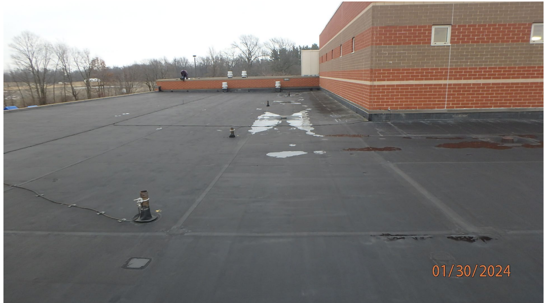
1.1.2.2 View of a line of roof drains on Roof Area B showing there is no significant ponding water. There is some minor ponding water near the roof drains. This can be corrected with addition of tapered insulation around the roof drains.
