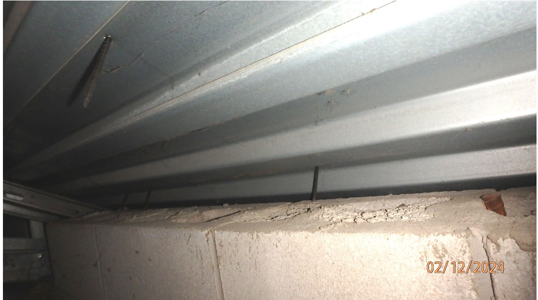
1.4.2.3 View of the same area from a different angle showing there is no air barrier installed at this location.
