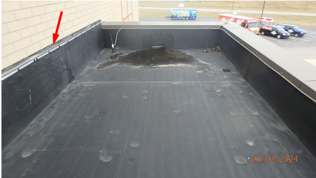
1.3.8 River Valley Middle School – View of an area where laminated copper flashing (red arrow) extends out of the wall.
