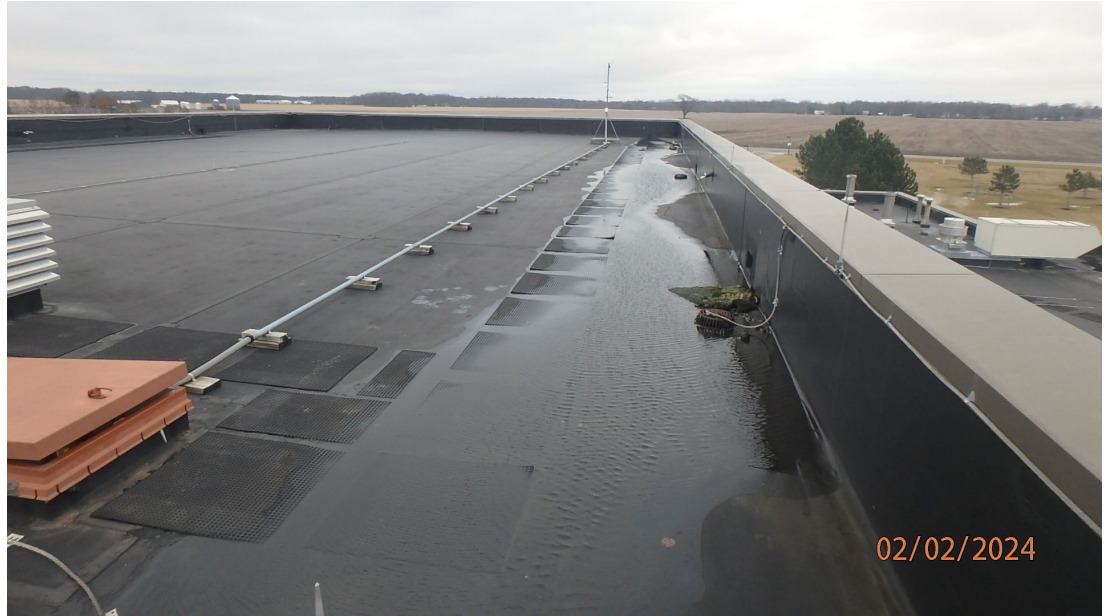
1.1.3.4 Overall view of the drain lines along Roof Area A showing there is significant ponding along the roof drain line that needs to be corrected. This can be reduced by the addition of tapered insulation around the roof drains and larger tapered insulation crickets.
