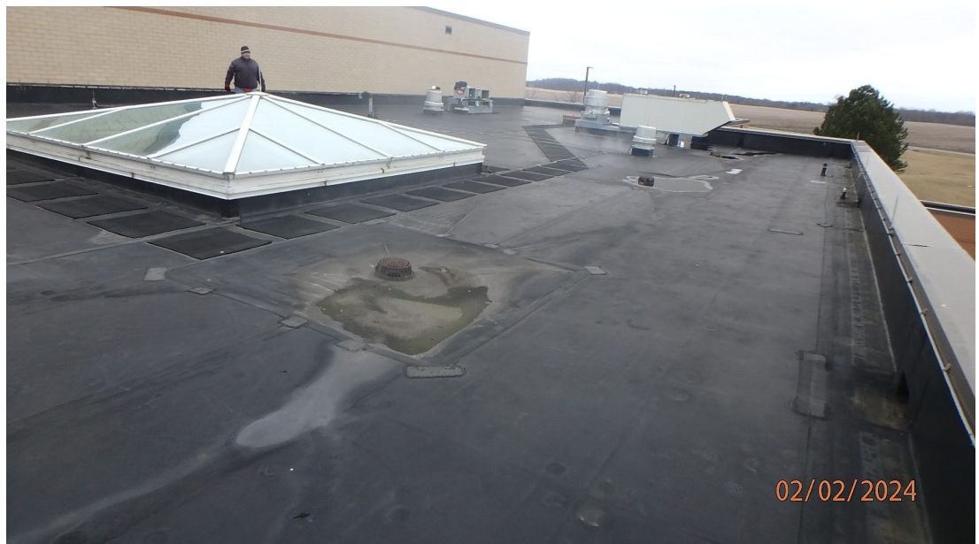
1.1.3.5 Overall view of the drain lines along Roof Area B showing there is some minor ponding around the roof that can be reduced by the addition of tapered insulation around the roof drains.
