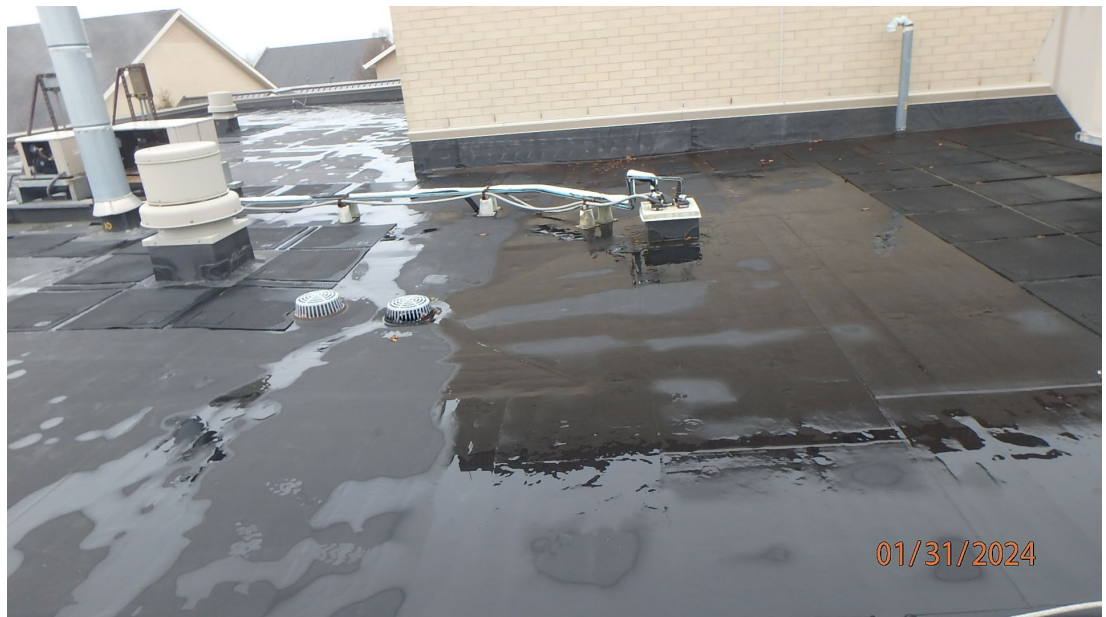
1.1.4.12 View of an area on Roof Area N showing there is no significant ponding on this roof area.
