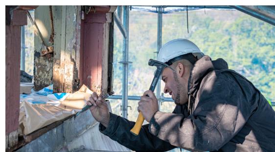
RESTORING THE CLOKKTOWER STRUCTURE
