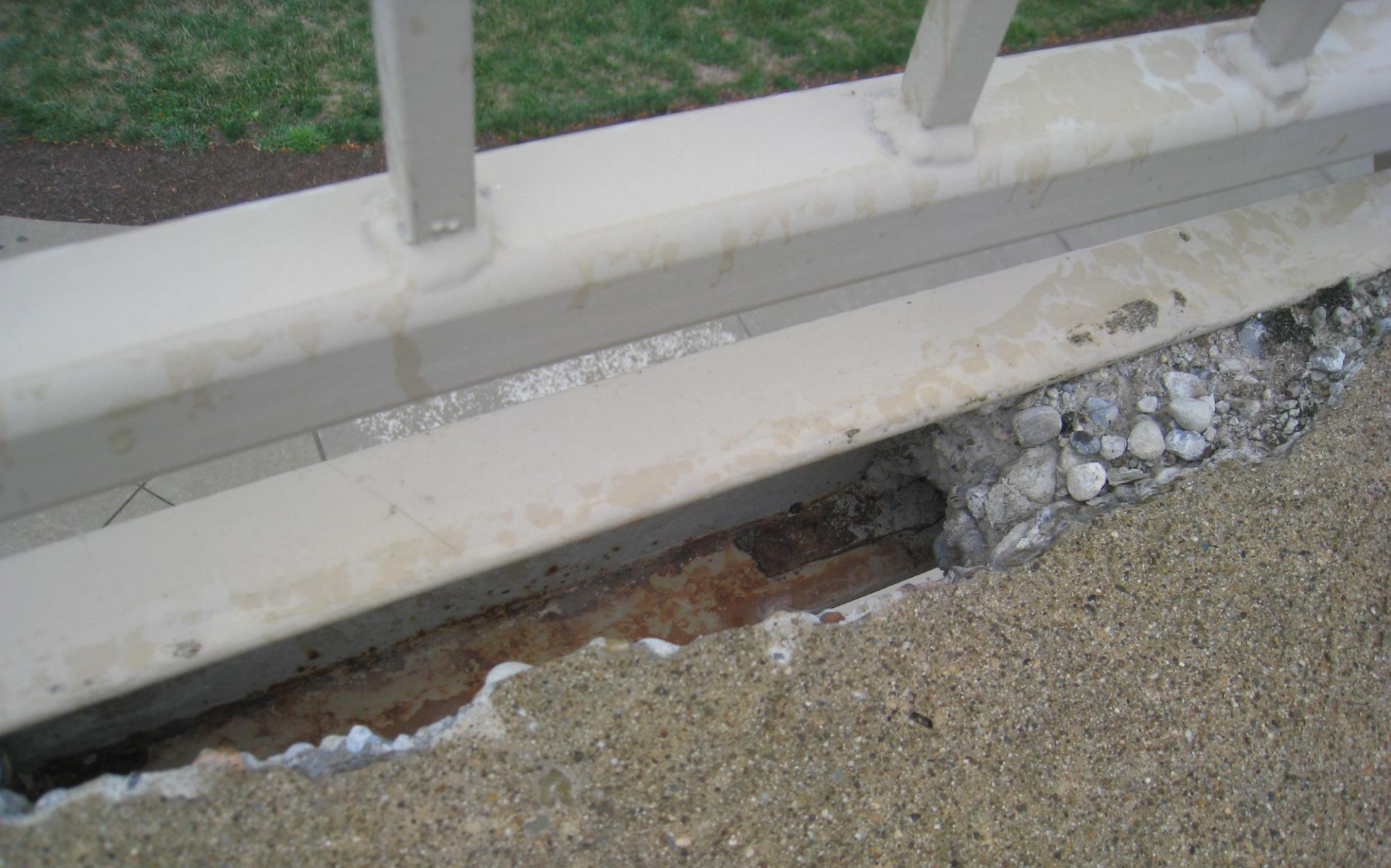
High School – Existing Pedestrian Bridge
