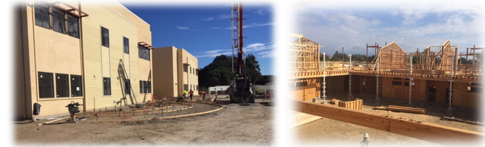
November 2017 Construction Progress at Lemonwood (Left) and Elm (Right)
