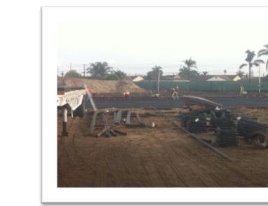
New Harrington Construction Site
