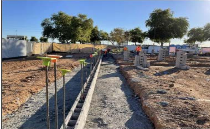
Masons laying 1 st course of stem.
