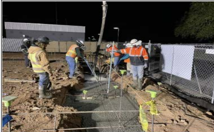
Pouring and checking footing heights.
