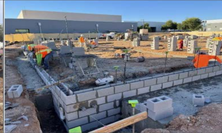
NE building corner step down footing and stem.
