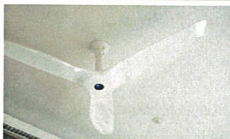
Ceiling height and oversize fans aid in ventilation and energy efficiency.
