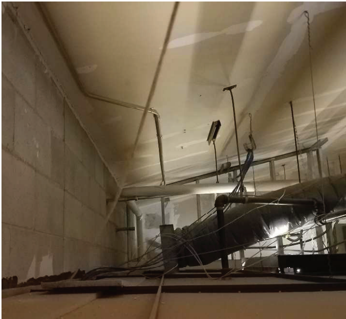
Fig. 6&7 – Interior ceiling plenum at exterior wall. The CMU to gyp is sealed but IR shows significant thermal leakage where the concrete meets the roof.
