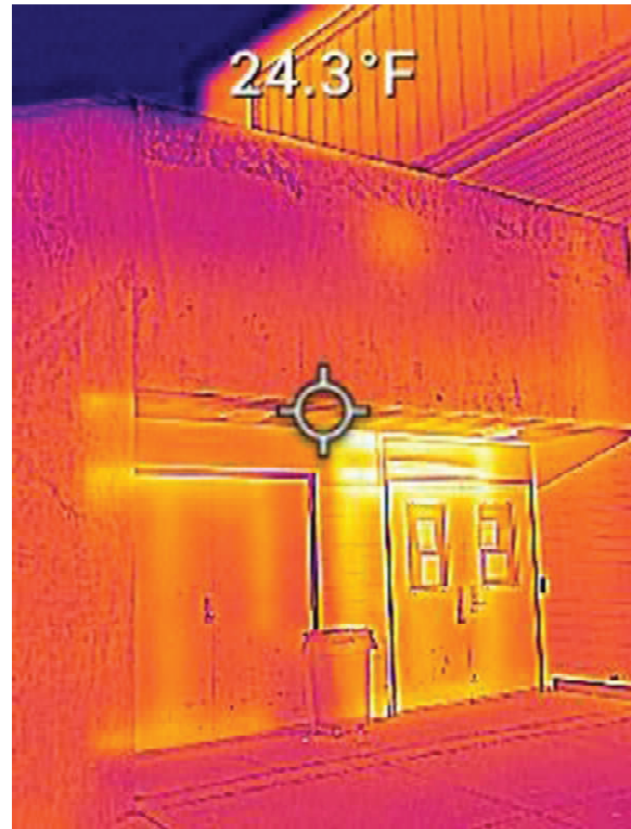
Fig.7&8 – SE Lower Entry – cast in place concrete structure with metal door frames. Heat signatures at frames and where concrete meets warm building envelope.s and where concrete meets warm building.
