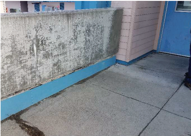
Fig.5&6 Classroom Entry, upper – flashing ok, thermal transfer at wall base.
