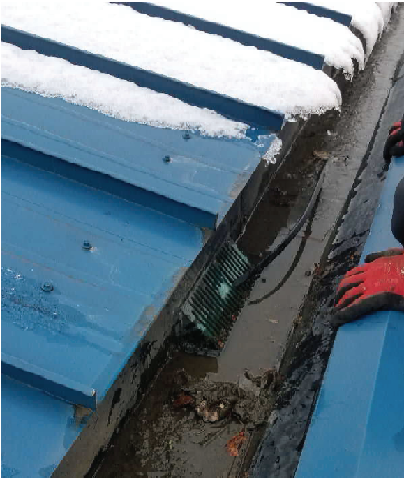
Fig.1 -North Gutter at Library – lot of silt
