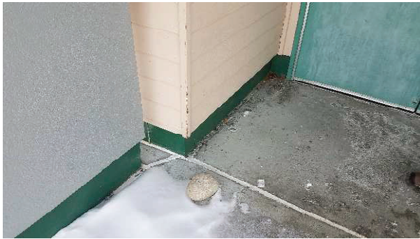
Fig. 10&11 SW upper Entry – flashing in ok condition along paving perimeter.
