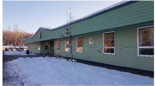
Fig. 12 Main Entry –siding discoloration and staining at valley, both sides of gable roof.
