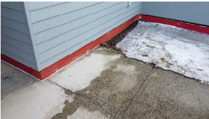
Fig.4&5 SW Upper Classroom Entry – some heat transfer at wall base. Open grade near overhang – has waterproofing degraded here?
