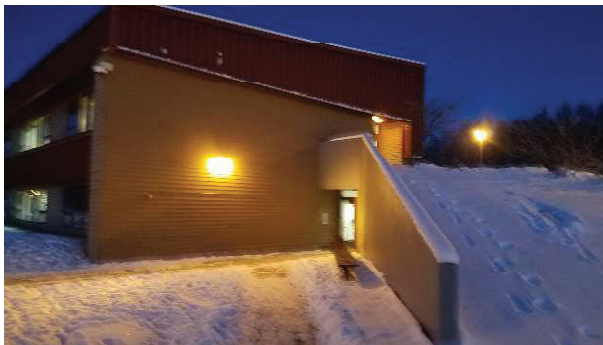
Fig. 4&5 – East entry lower level. IR shows some thermal leakage where the concrete meets exterior wall.Metal door and frame are also a big thermal transfer.
