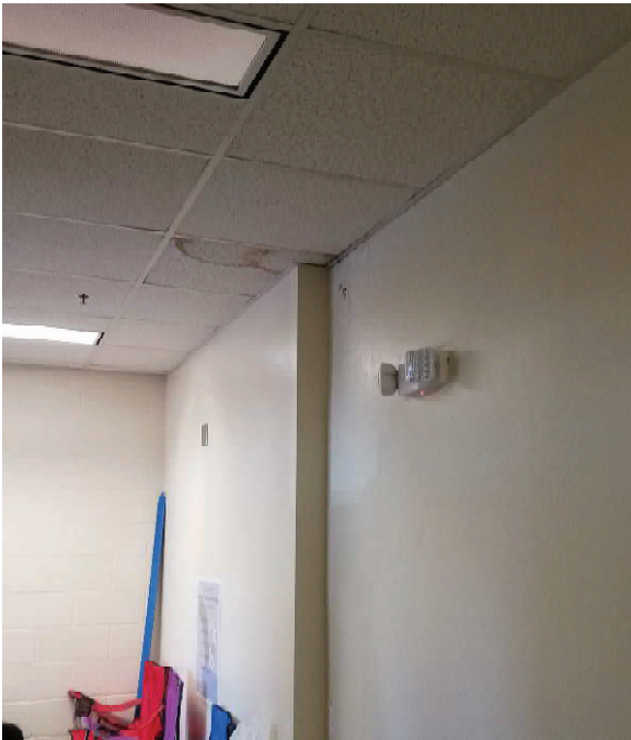
Fig. 5&6 – Interior ceiling plenum at SW lower Entry. This is the inside corner at the wall jog above. There is leaking, stained ceiling tiles, and what appears to be a spray applied leak sealant applied in the plenum. There is also IR leakage and evidence of air leakage in this area.
