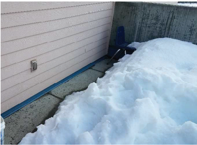
Fig.7&8 Classroom Entry, upper – flashing ok, thermal transfer at wall base.
