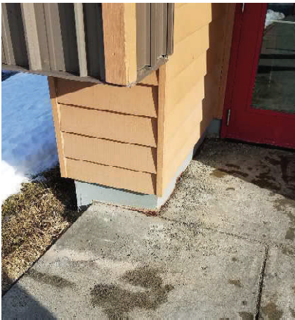
Fig.2&3 Upper SE Classroom wing Entry – some corrosion at flashing.
