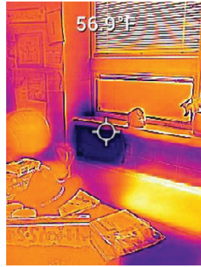
Fig.11&12 Upper SE Classroom Window – area of leakage has noticeable darker areas. This indicates damaged insulation.
