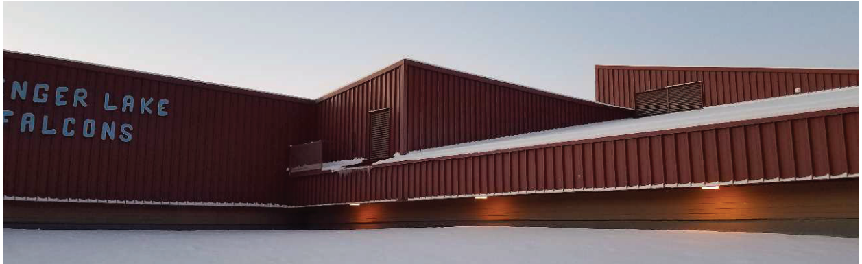
Fig.1 -North Gutter at Library – even snow cover.Mech Louver melts snow at roof edge.
