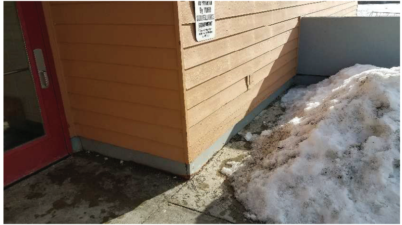
Fig.2&3 Upper SE Classroom wing Entry – some corrosion at flashing.
