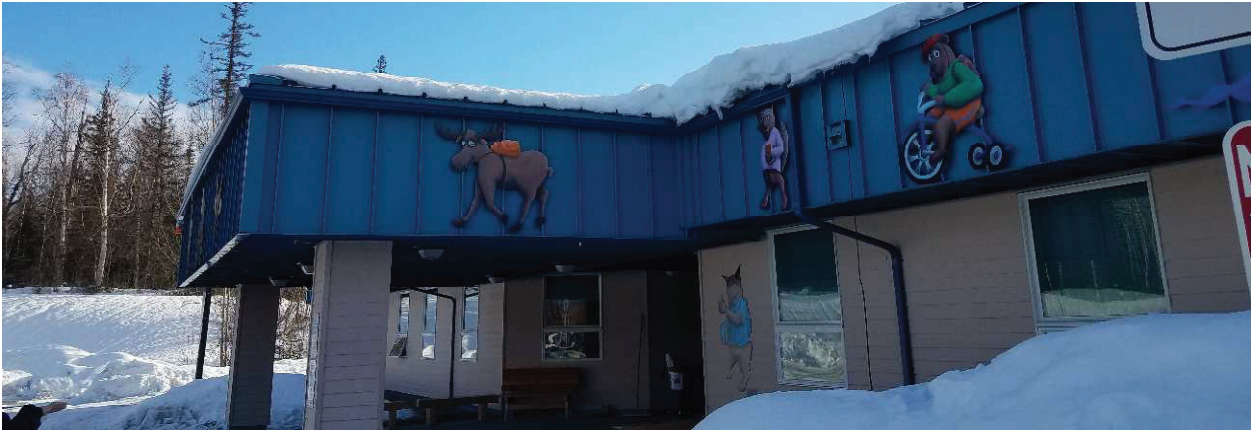
Fig. 1 Main Entry –slopes back towards building and seasonally floods over.
