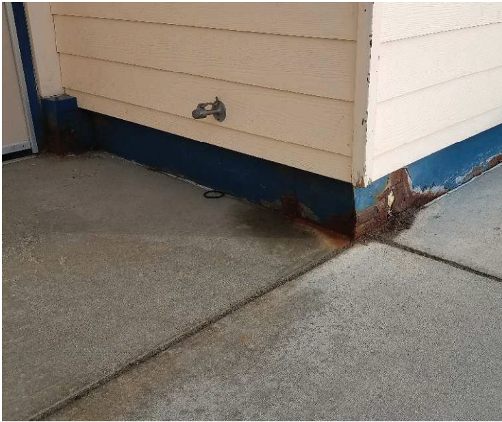
Fig.11&12 – SE Entry, upper landing – Metal edge flashing pulled away and corroded. Definite heat loss along this edge.
