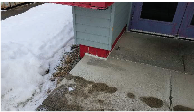
Fig.2&3 SW Upper Classroom Entry – some heat transfer at wall base.
