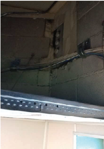
Fig. 3&4 Interior ceiling plenum at Front Desk – heat loss at beam pocket.
