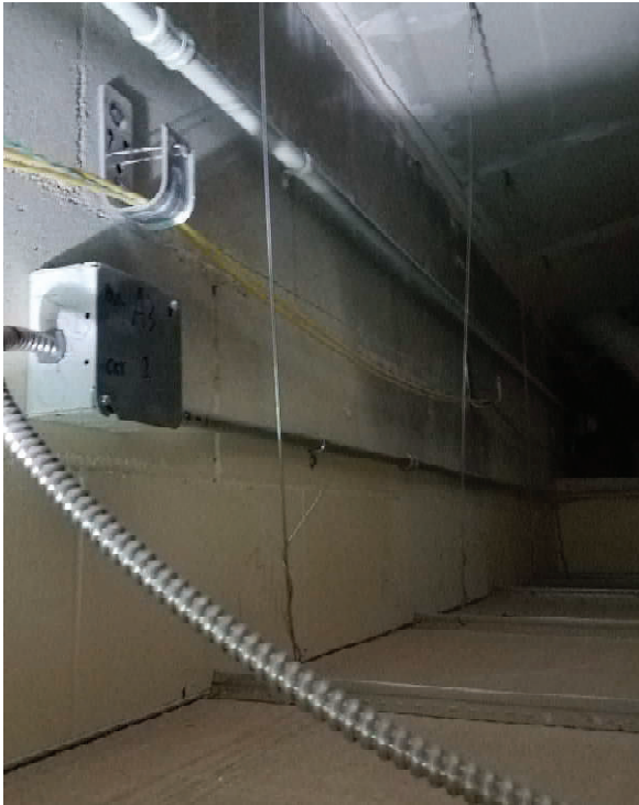
Fig.6&7 – Interior ceiling plenum at exterior wall. Gyp sealed to CMU wall. Some penetrations. Cold spot at the top of the wall, but not enough to condense.
