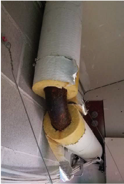
Fig. 7&8 Interior ceiling plenum at Classroom, north wall – leak area at rain leader has insulation removed. No heat trace.
