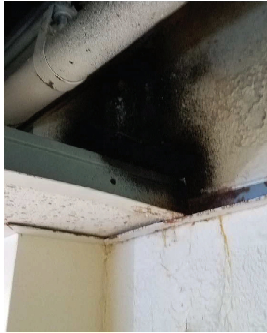
Fig. 5&6 – Interior ceiling plenum at SW lower Entry. This is the inside corner at the wall jog above. There is leaking, stained ceiling tiles, and what appears to be a spray applied leak sealant applied in the plenum. There is also IR leakage and evidence of air leakage in this area.
