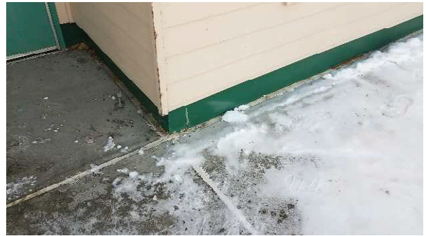
Fig. 10&11 SW upper Entry – flashing in ok condition along paving perimeter.
