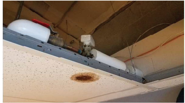
Fig. 2– Interior ceiling plenum at exterior wall, Staff Break Room. Leak at hydronic control valve actuator.
