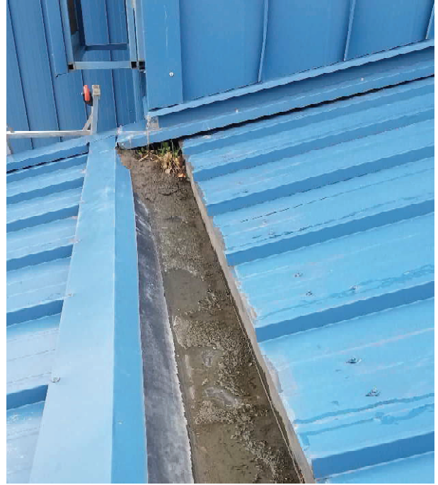
Fig. 2 - North Gutter at Library, looking East – silt
