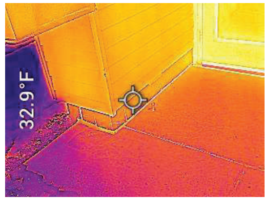
Fig.2&3 SW Upper Classroom Entry – some heat transfer at wall base.
