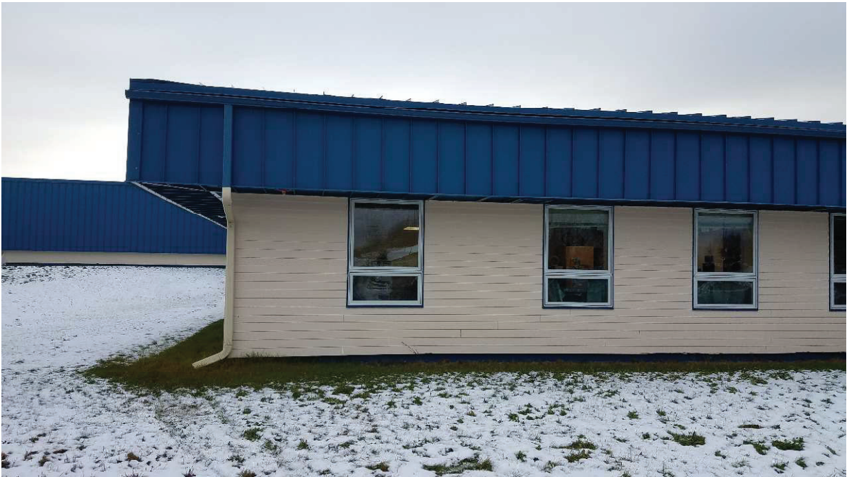
Fig.5 -NW corner, exterior gutters and downspouts at eave.Note that these are in addition to the internal gutters that occur just over the exterior walls.
