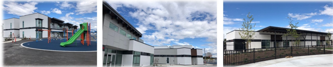
Reconstructed McKinna Elementary School
