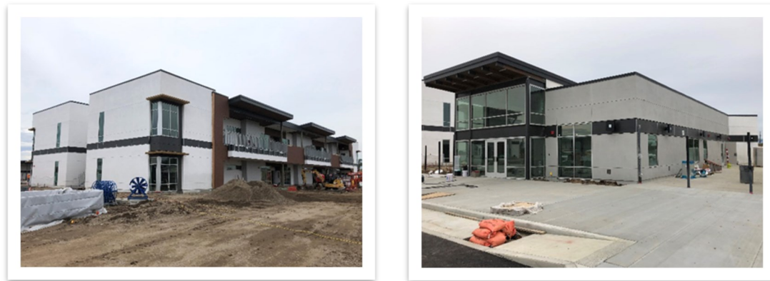
New Classroom Building and Administration Building—Construction Progress
