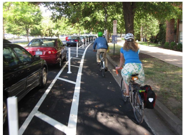
Figure 9-12: Parking buffered bike lane with traffic delineator posts. Source: League of American Bicyclists
