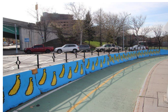
Figure 9-8: Decorated concrete barrier with steel railing. Source: Curbed New York
