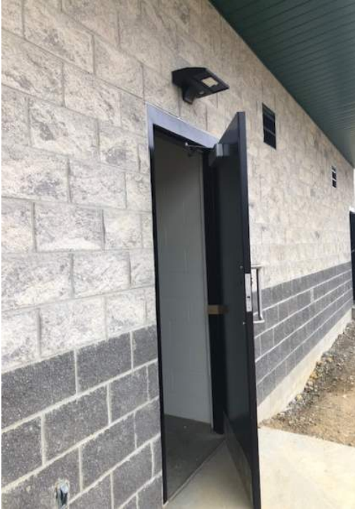
05.14.24 - Exterior Light Fixtures at Concession Stand
