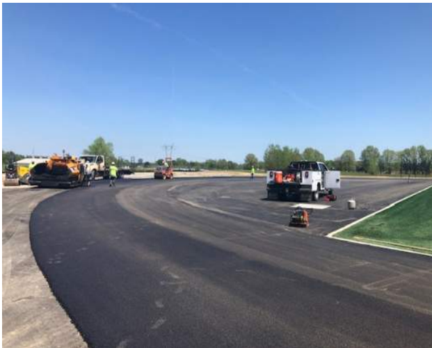
05.02.24 - Asphalt Paving at Track - Surface Course
