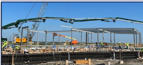
Progress in Area C.
